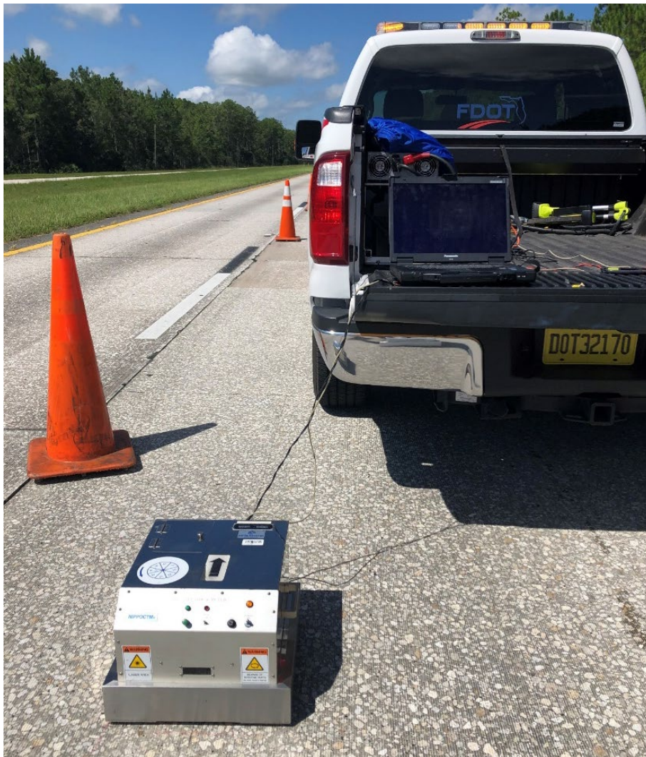
Figure 5-3. CTM at an LGD concrete test site.
