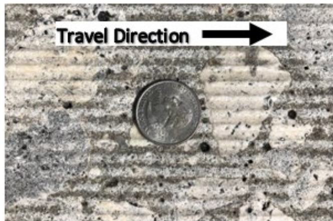
Figure 5-12. Longitudinal texture of concrete roadways in Florida.
