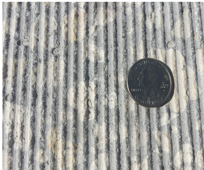
Figure 2-21. Diamond ground concrete road [26].
