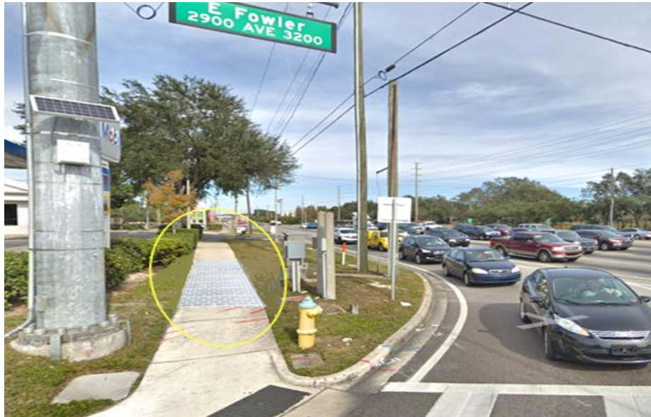
Figure 15. Solar roadway panels on sidewalk near traffic signal cabinet
