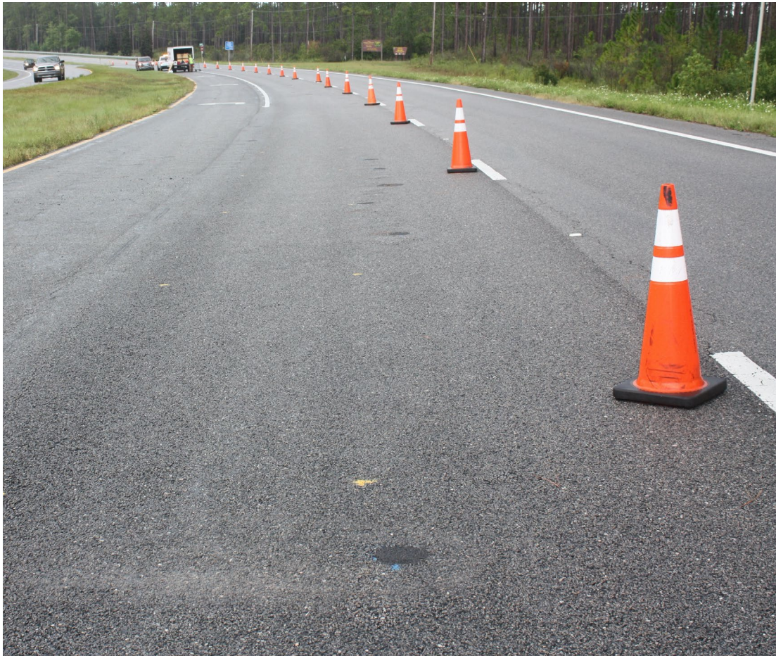
Figure 3-3. SR 79 Roadway Overview
