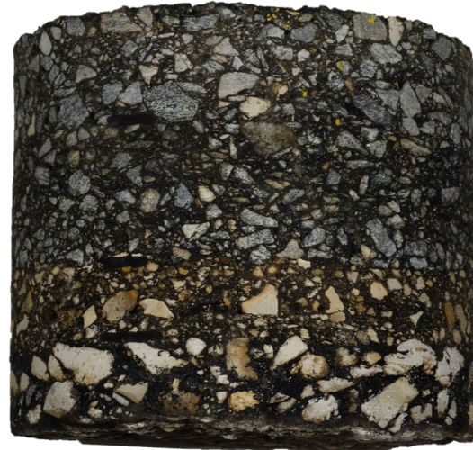
Figure 4-60. SR 24 Typical Control Section Core at MP 22.489
