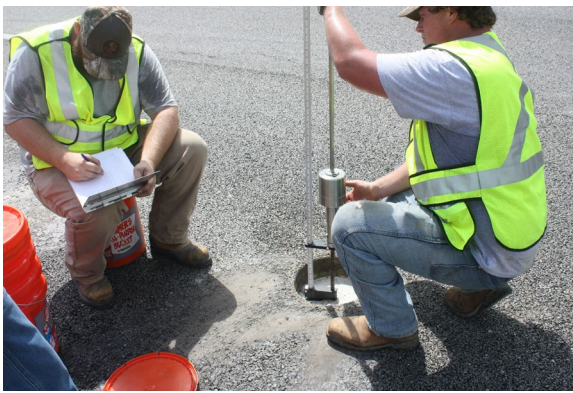
Figure 3-22. Manual DCP Test
