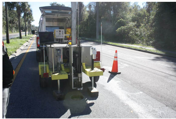
Figure 3-23. Automated DCP Test
