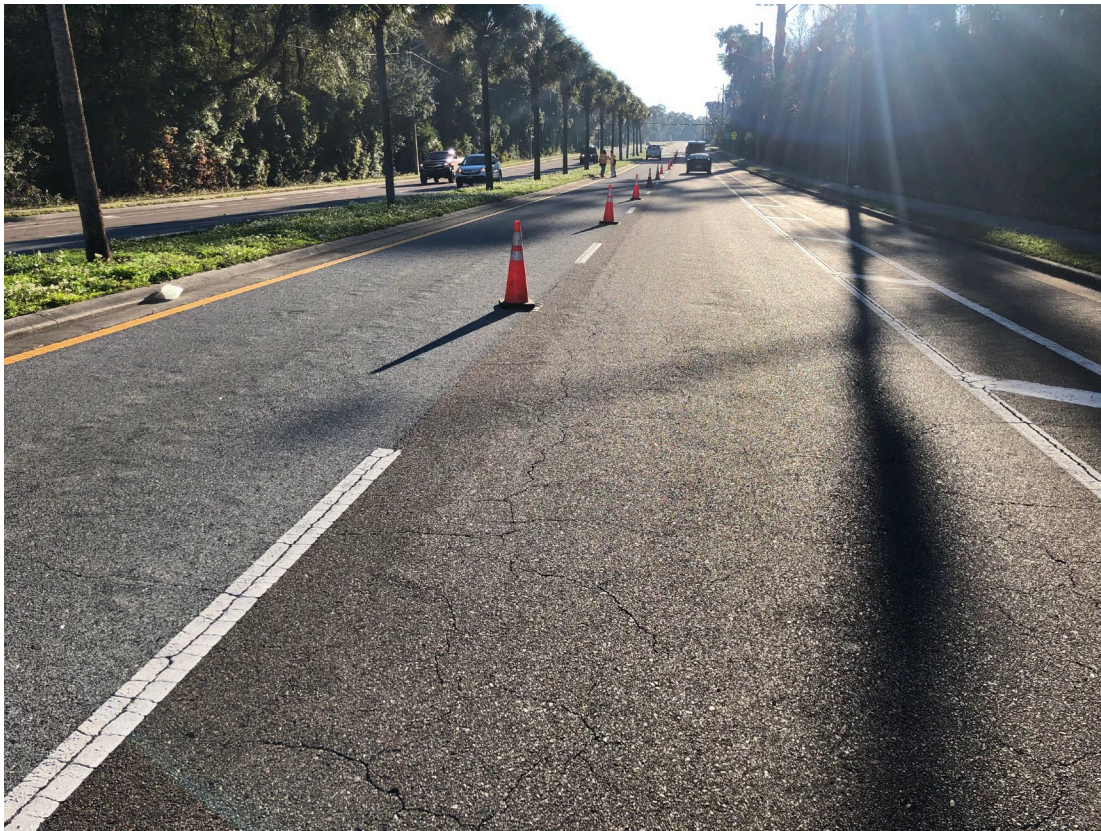
Figure 3-11. SR 20 Roadway Overview
