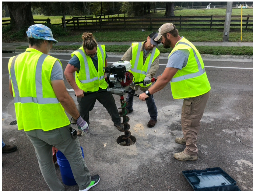
Figure 3-21. Sampling Base, Subgrade, and Embankment Materials
