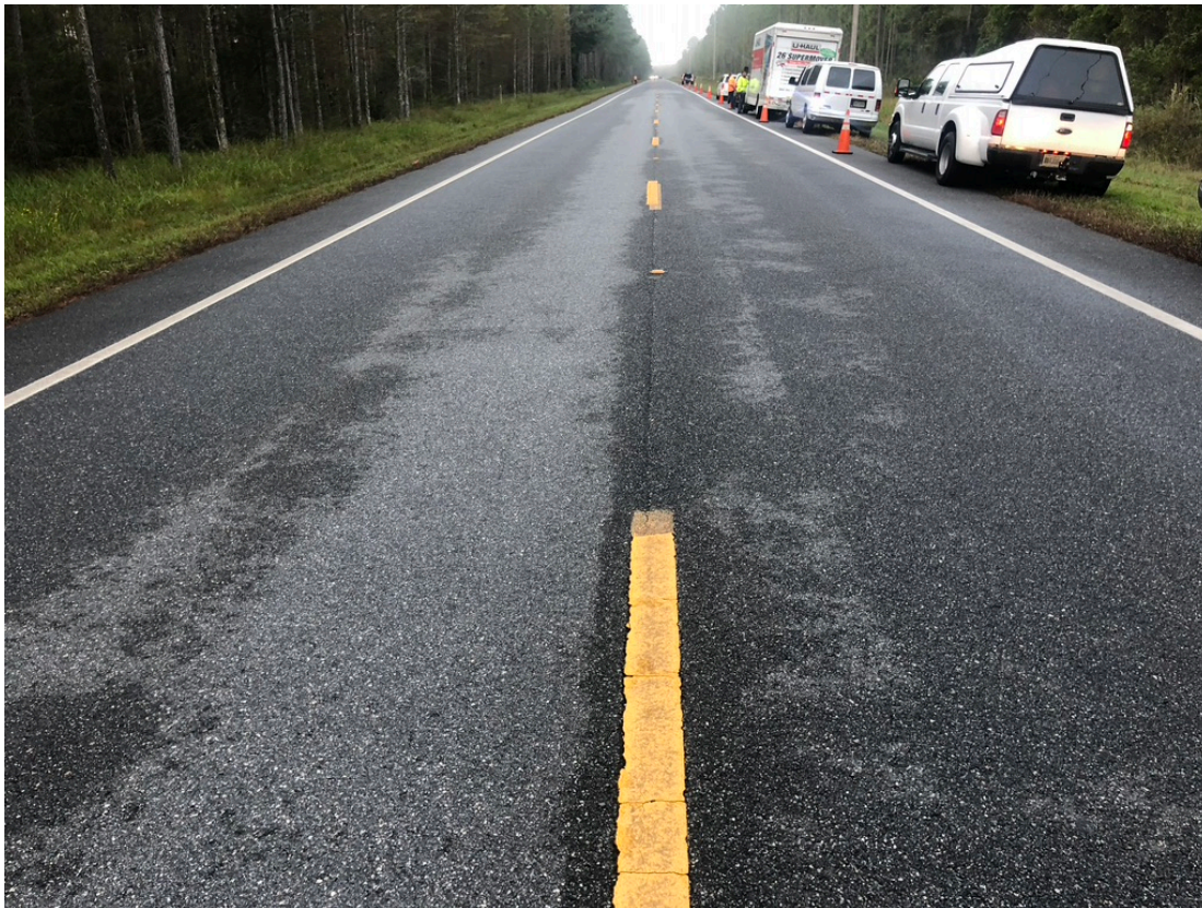
Figure 3-7. SR 24 Roadway Overview
