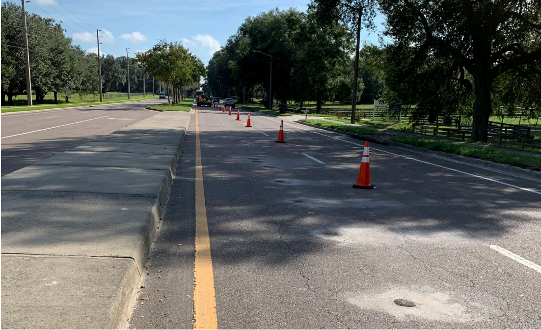
Figure 3-5. SR 26 Roadway Overview
