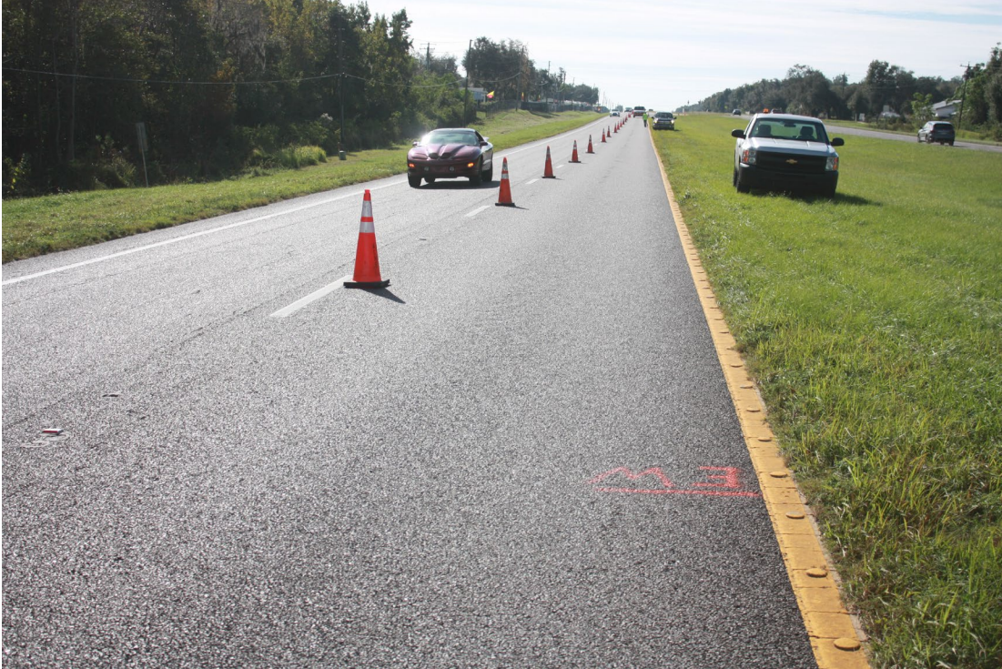
Figure 3-9. US 17 Roadway Overview
