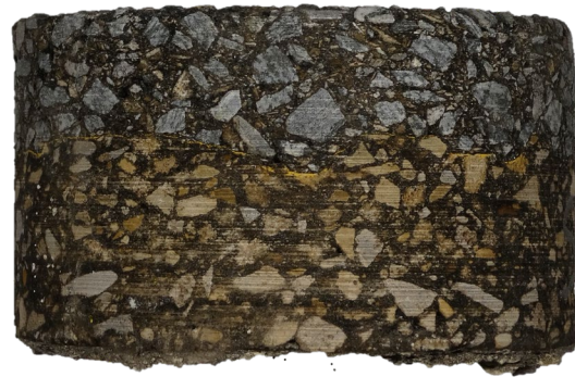
Figure 4-70. SR 24 Typical Control Section Core at MP 2.931
