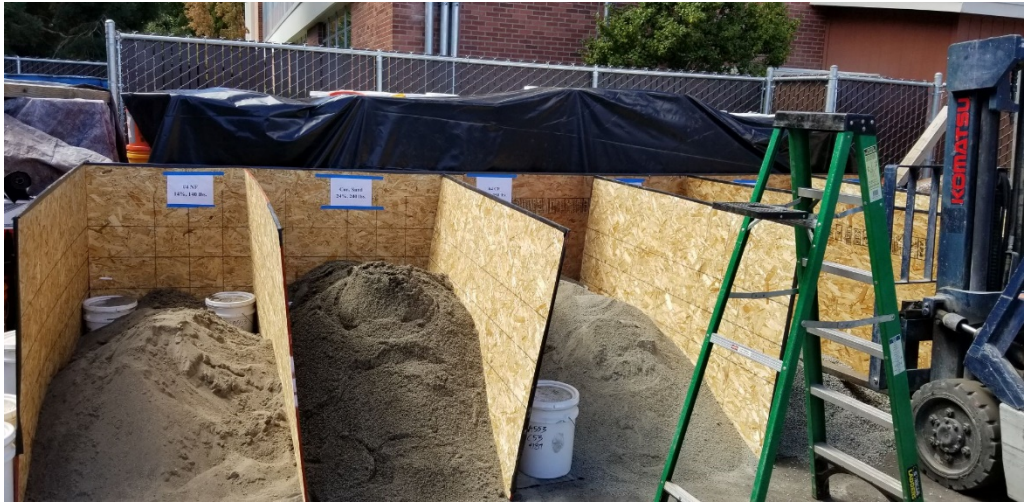
Figure 7-28. Aggregate stockpiles organized and used to produce PMA and HP AC mixes.
