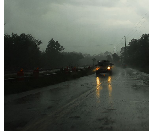
With Florida's frequent rain, the superior drainage of open-graded friction courses is valuable, especially if their durability can be improved.
