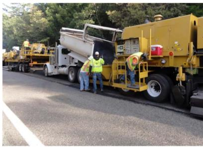
Figure 16. Addition of New Hot Mix (photo courtesy of ARRA)
