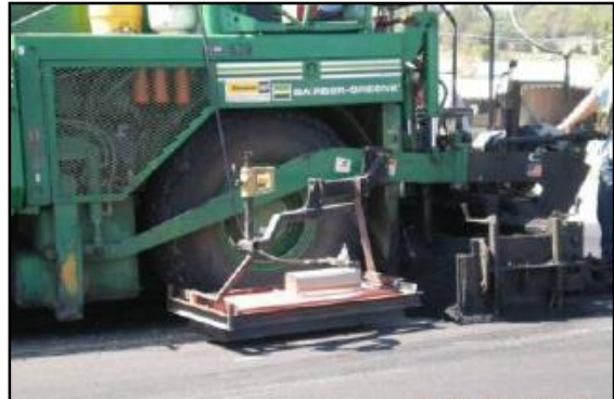
Infrared joint heaters improve joint density.
