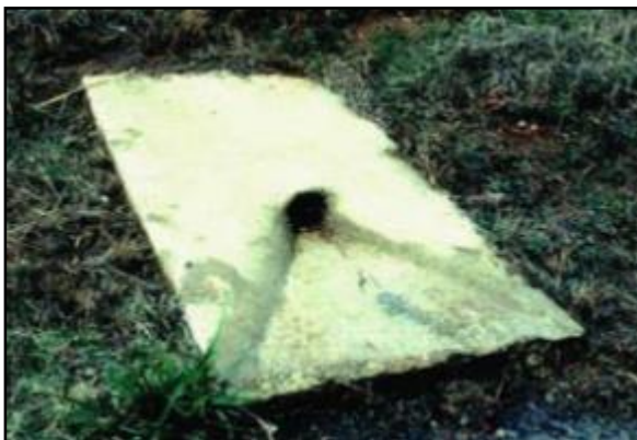
Painted arrow reference marker to aid locating drain outlets.
