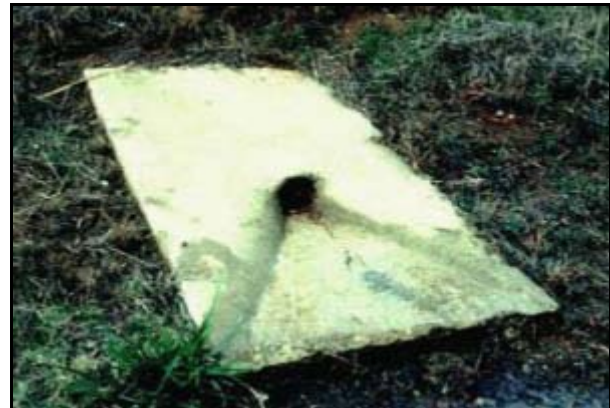
Figure 23. Large headwall for outlet pipe.
