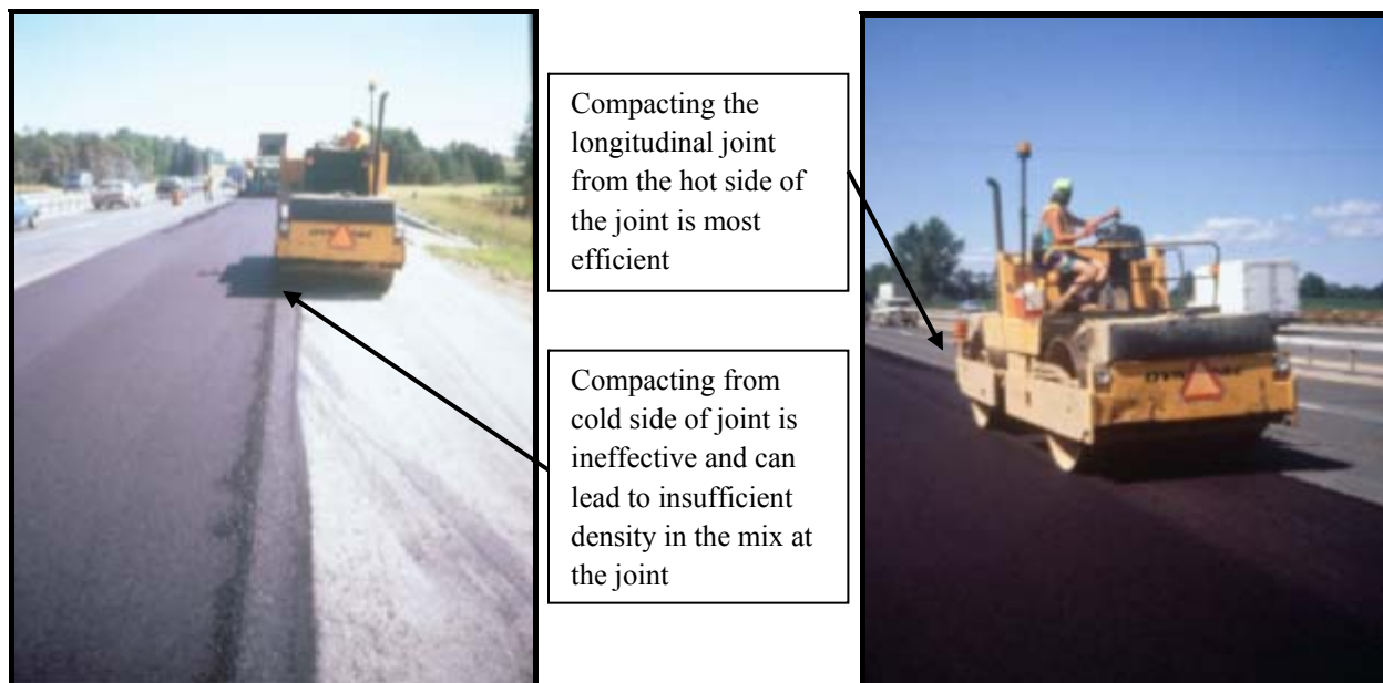
Figure 8. Techniques for compacting HMA longitudinal joints.
