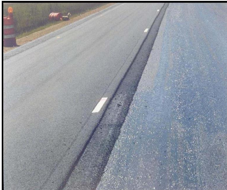
Figure 8. Notched wedge joint.
