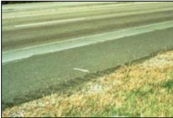
Painted arrow reference marker to aid locating drain outlets.
