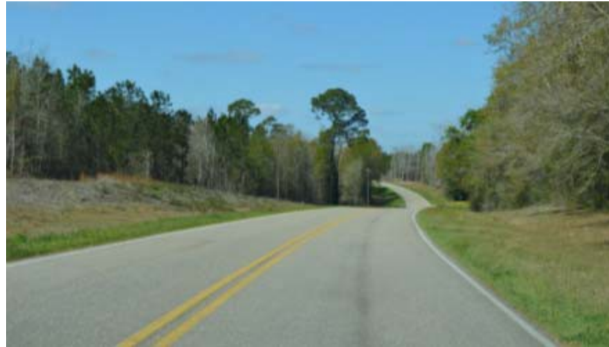
Flexible pavement section in good condition.
