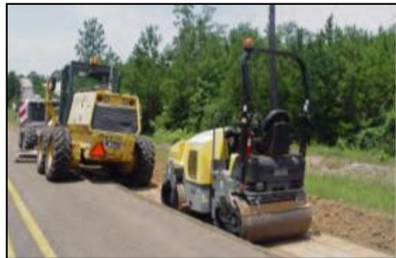
Compacting narrow widening sections
