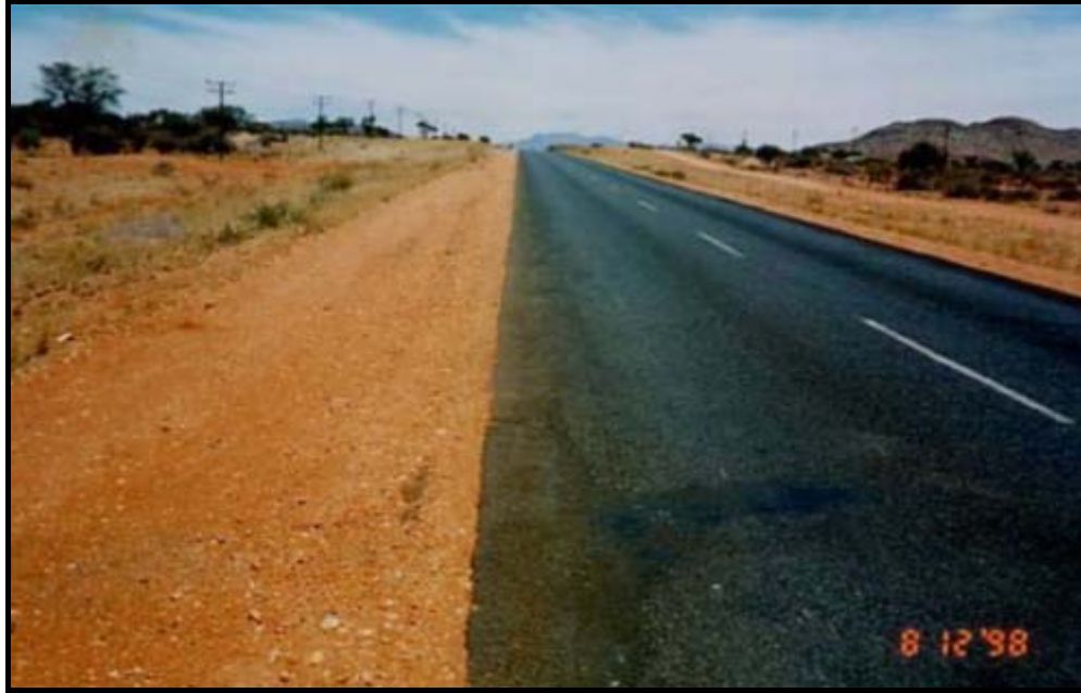
Figure 39. Finished edge widening overview.
