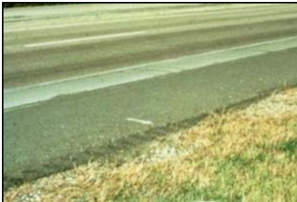
Figure 22. Painted arrow reference marker.
