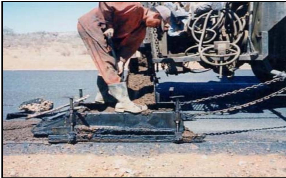
Figure 38. Coarse-graded slurry placement.
