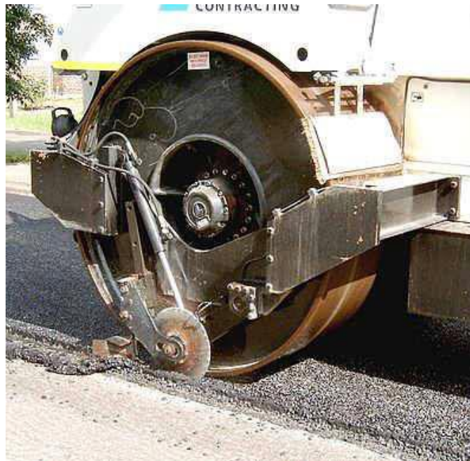
Figure 5. Cutting wheel removing approximately 2 inches of material along cold lane.
