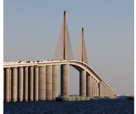
Repairs made with GFRP concrete reinforcing bars to the sea walls along the Sunshine Skyway Bridge Rest Area will reduce the need for future repairs.
