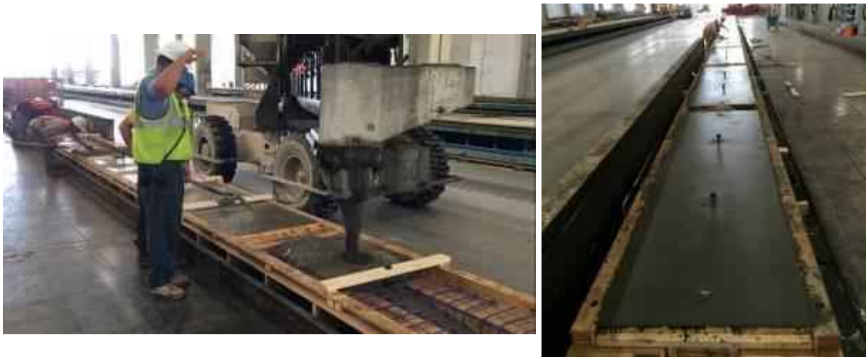
Figure 6.7: Casting of Concrete
