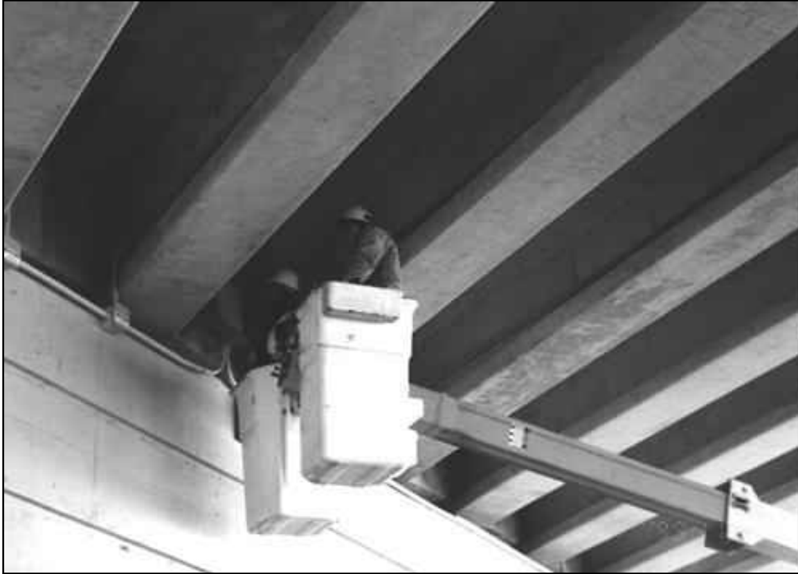
Figure 2.28: Beddington Trail Bridge, Calgary, Canada (ISIS Canada, 2009)
