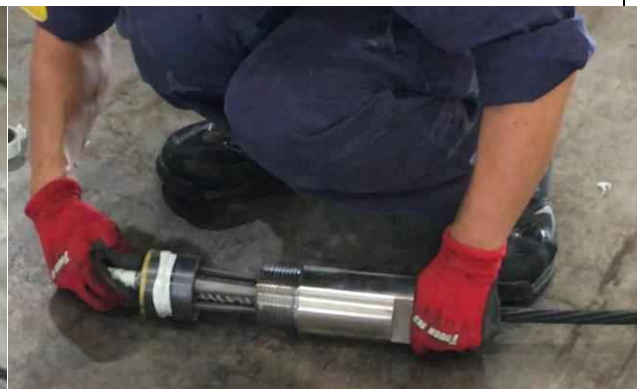
(f) Placing wedge guide into the CFRP sleeve
