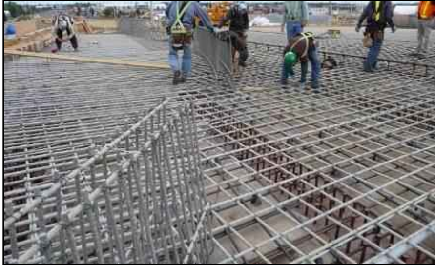
(b) FRP decks and barriers – Gateway Blvd/23 rd Ave – Alberta (2009)
