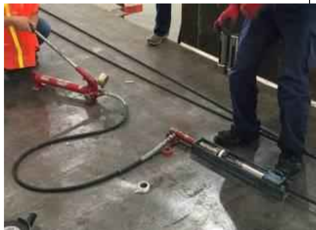
(h) A hand pump presses the wedges into the sleeve
