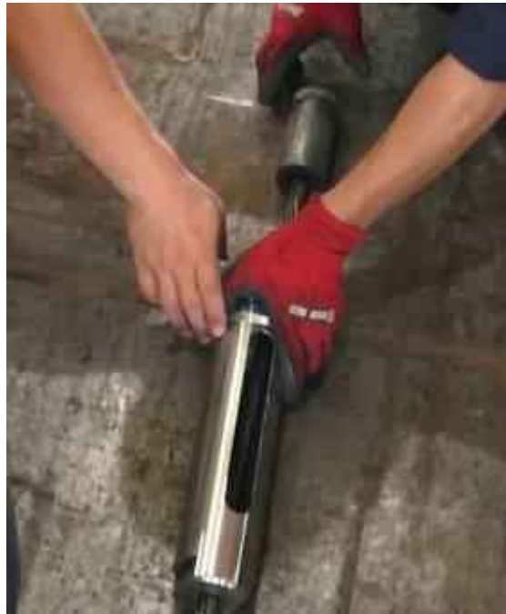
Figure 6.3: Preparation of steel strand part of the coupler
