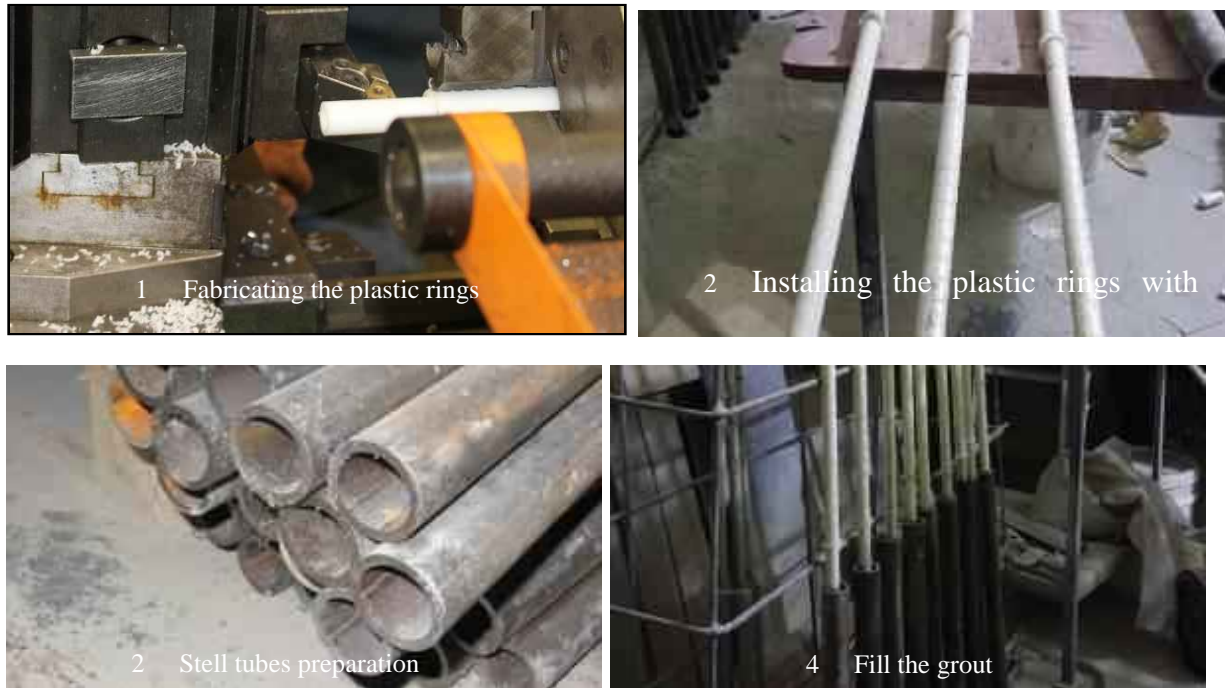
Figure 4.4: Preparation of the test GFRP bar specimens
