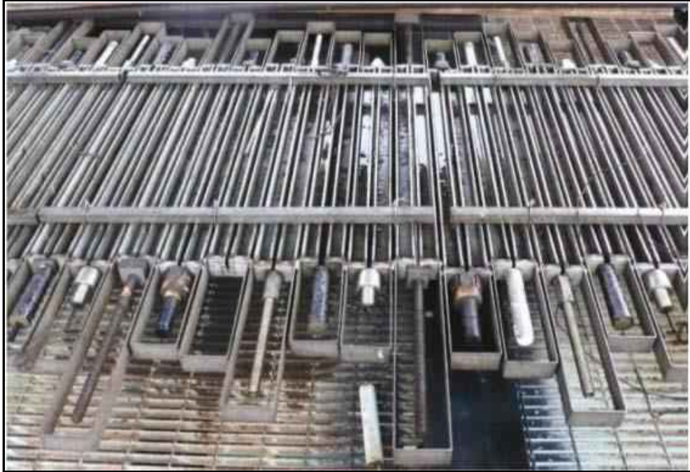
Figure 2.18: FRP cables pre-stressed in SUS flames (Sasaki and Nishizaki 2015)
