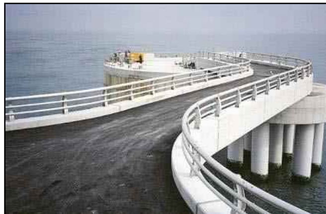
Figure 2.25: Haranomachi thermal power plant outfall Bridge
