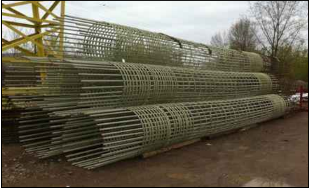
(a) Overview of the GFRP soft eyes
