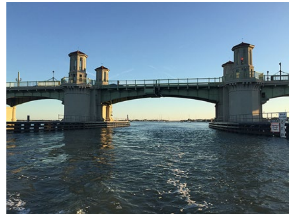
Structural plastic can be used to protect bridge elements, like the fenders on this historic bridge, from marine vessel impacts.
