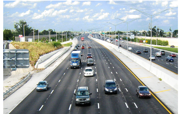
The inner lane on this stretch of I-95 in Florida is an HOV lane, separated from the general purpose lanes by double lines and a three-foot buffer.
