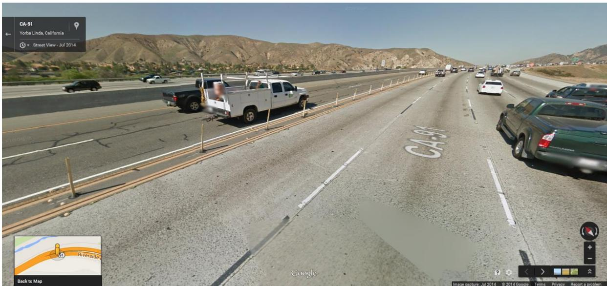
**Figure 3.13 HOT Lane Separation on California SR-91**
