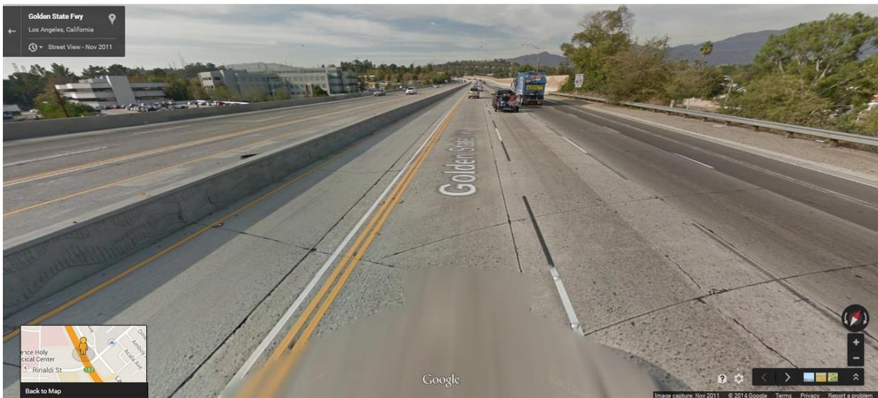
**Figure 3.4 California Buffer Separation on I-5 (Buffer of 1-2 feet)**
