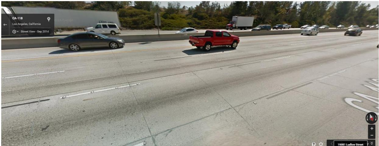
**Figure 3.2 California Buffer Separation on SR-118 (Buffer of 1-2 feet)**
