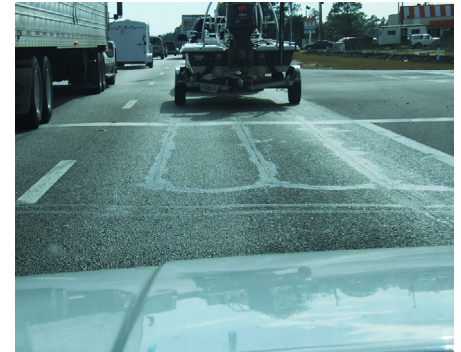
Detector loops track the presence of vehicles and can be a valuable source of traffic data.
