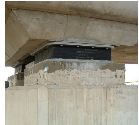
Bearing pads allow massive bridge parts to safely move under the influences of traffic loads and temperature.
