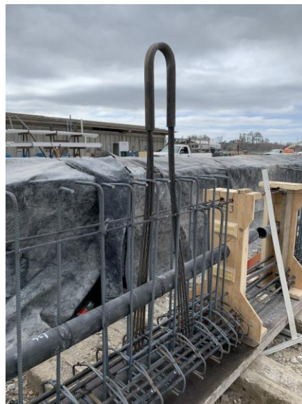
Figure 5.10 Lifting loops for transportation
