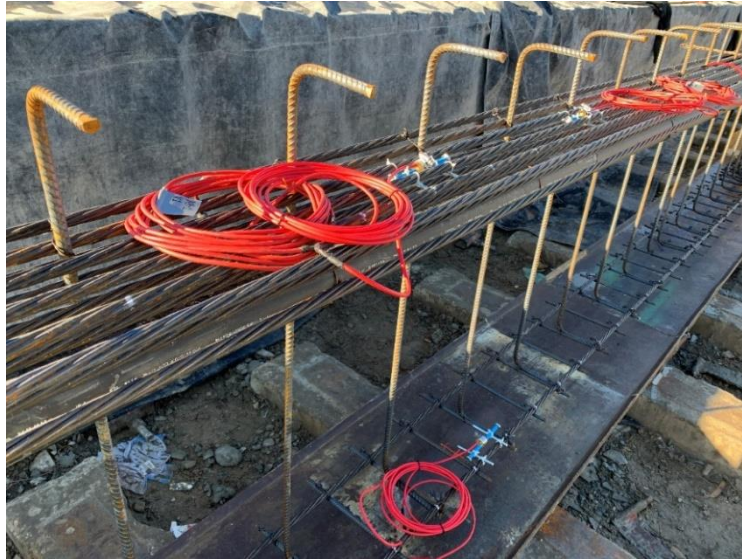
Figure 7.20 Vibrating wire gages installed in NB precast specimens
