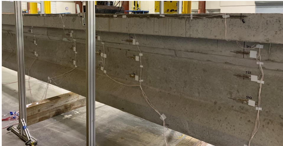
Figure 5.31 Typical 60-mm foil strain gages installed on SS precast specimens
