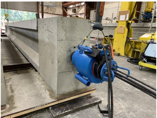
Figure 5.23 Post-tensioning of precast SS specimen
