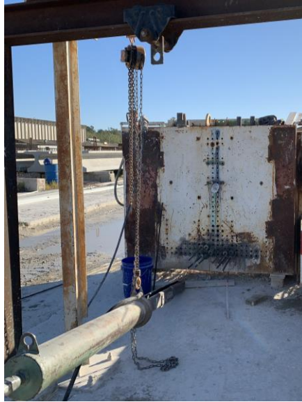
Figure 5.5 Prestressing strands at live end and monostrand hydraulic jack
