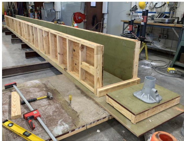
Figure 6.1 Plywood formwork used in the fabrication of CIP specimen SS-5
