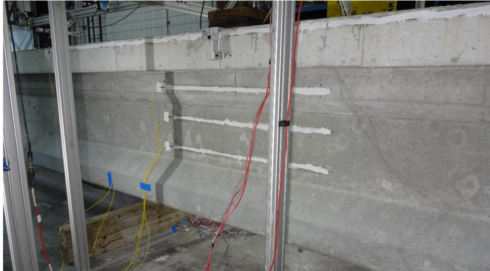
Figure 5.33 Typical fiber optic sensors installed on SS precast specimens
