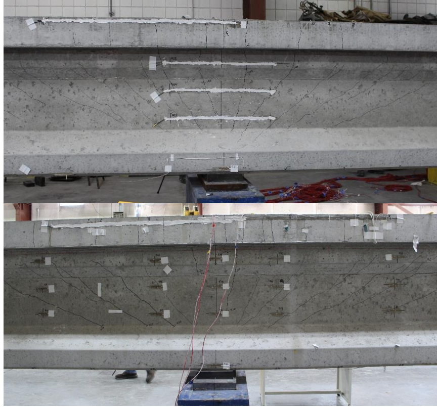
Figure E.1 Beam specimen NB-1 at end of testing: (a) East side (fiber optic sensors) and (b) West side (foil strain gages)
