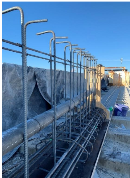
Figure 5.8 Rebar cage for SS specimen
