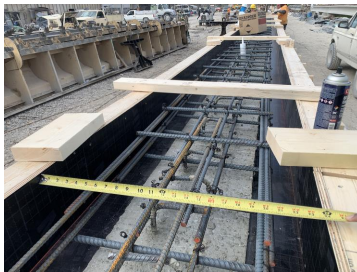
Figure 5.13 Mild steel reinforcement for concrete deck
