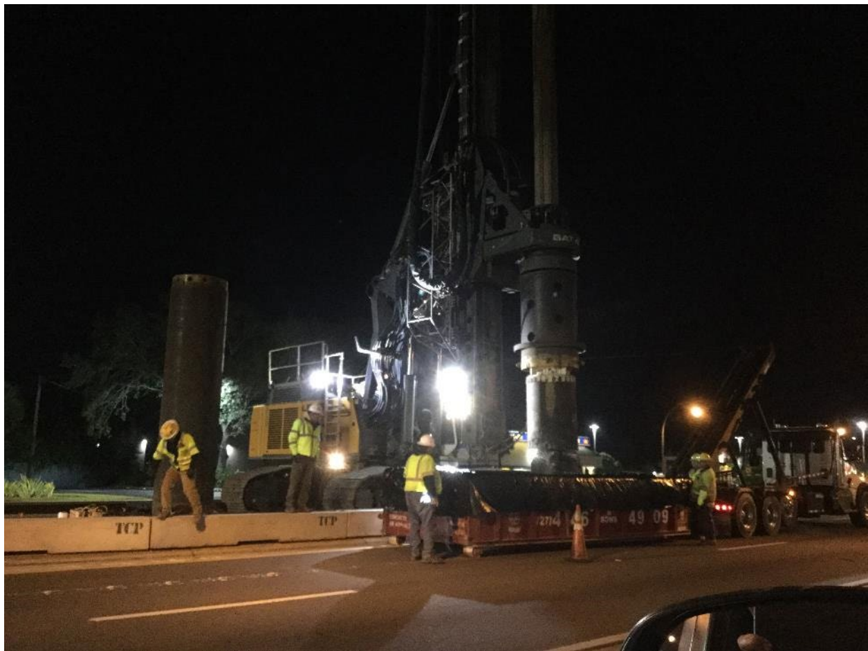
Figure 2-9. Drilling Test Shaft 3.
