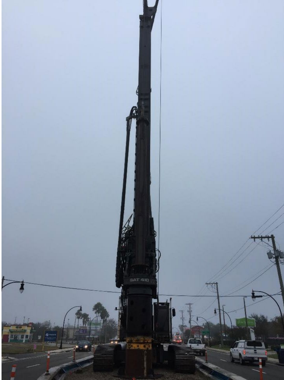
Figure 2-2. Liebehrr BAT 410 drill rig.
