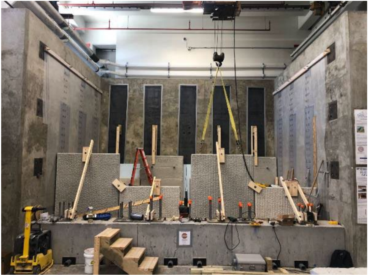
Figure 4-13. First course of MSE wall panels completed.
