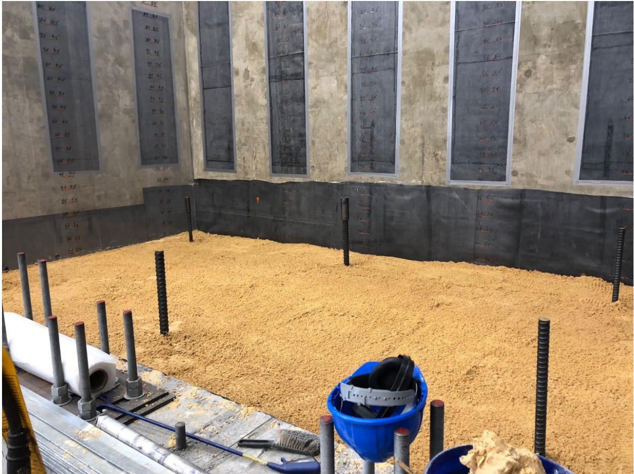
Figure 4-6. Base layer soil placement.
