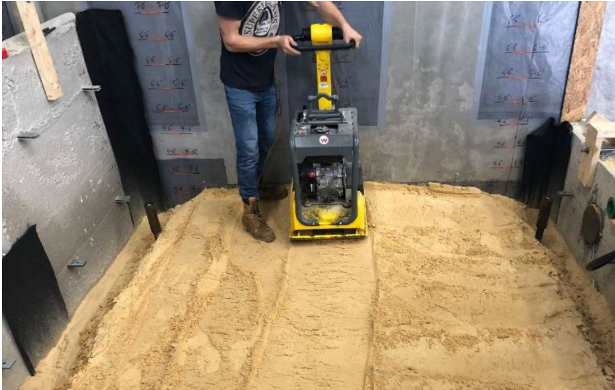
Figure 4-21. Soil compaction prior to installing the first row of reinforcement strips.
