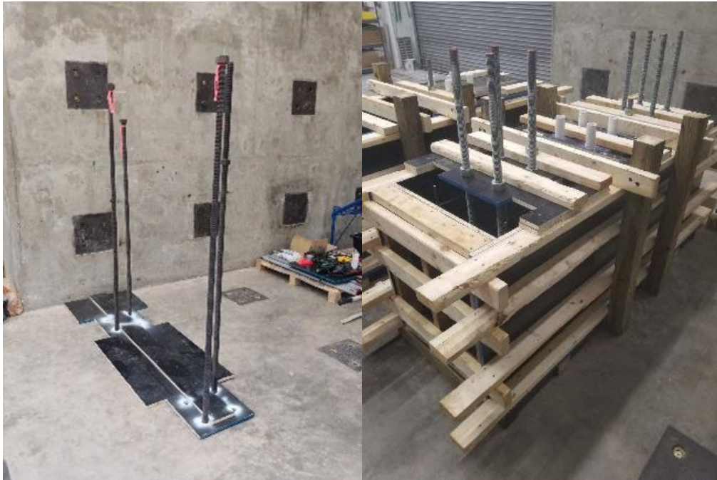
Figure 4-1. Constructing forms to cast base layer retaining concrete blocks.
