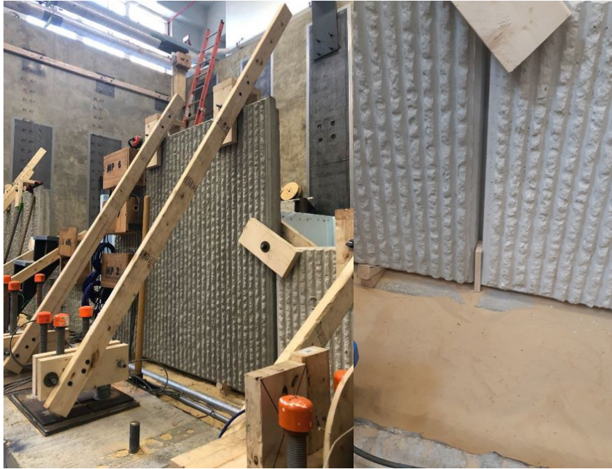
Figure 4-28. Temporary wall bracing, spacers, wedges, and clamps in place.
