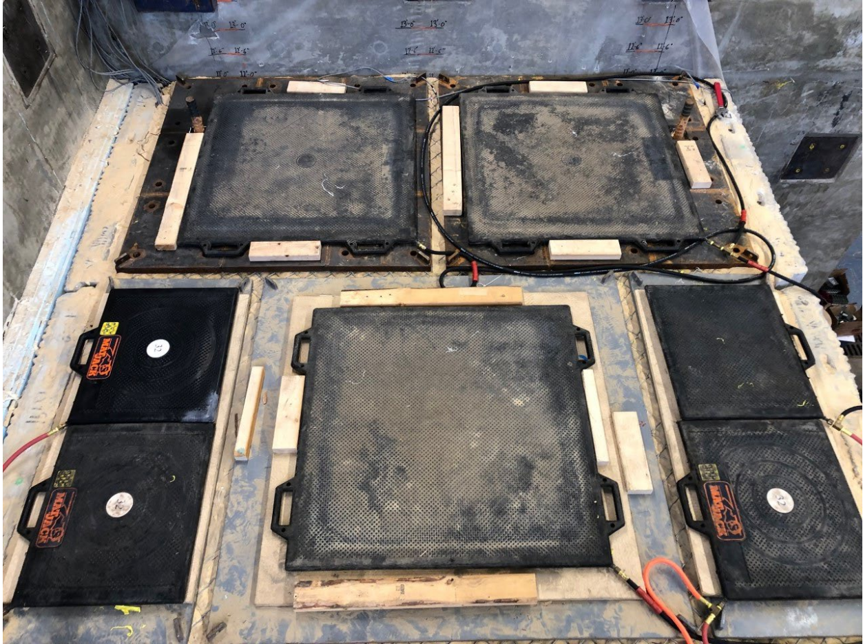
Figure 4-35. Matjack airbag system in place on the 103% compaction effort side.
