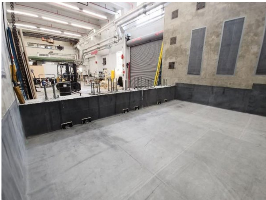
Figure 4-3. EPDM rubber placed throughout the research area to protect metal tie-ins.
