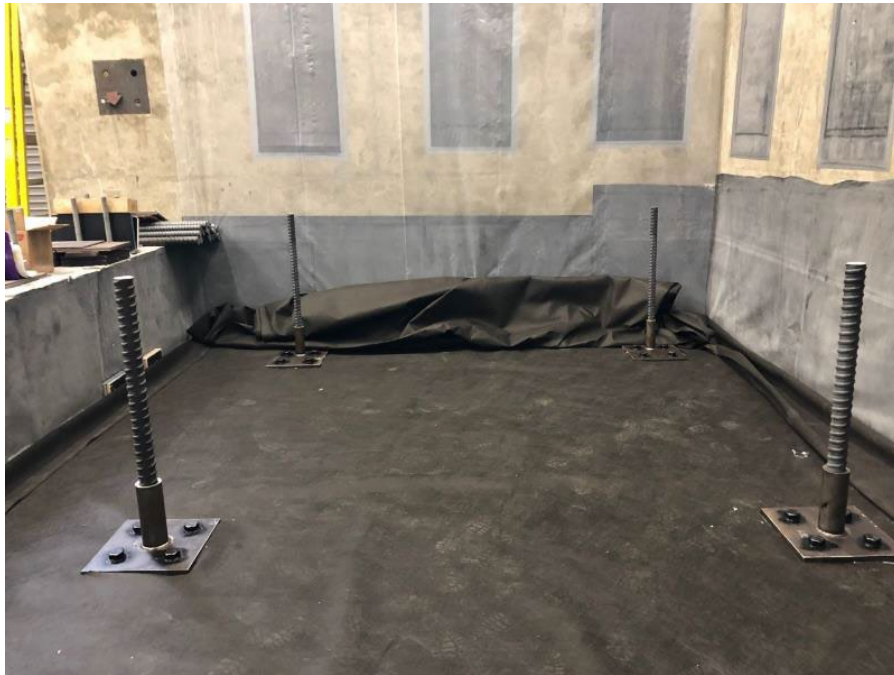
Figure 4-4. Structural geotextile placed and threaded rods mechanically fastened to strong floor.
