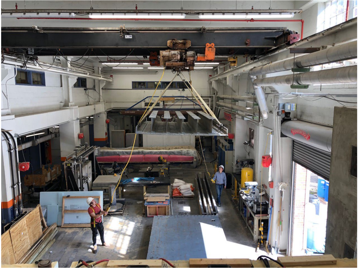
Figure 4-36. Crane lifting the first soil box wall in place.
