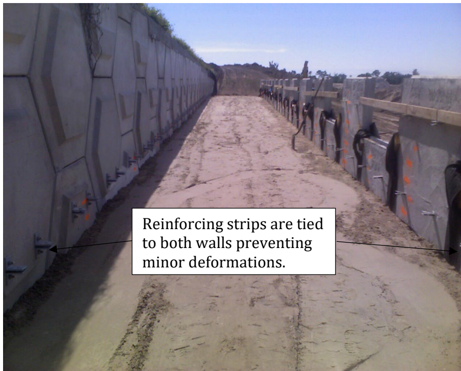
Figure 1-2. MSE wall embankment widening scenario.
