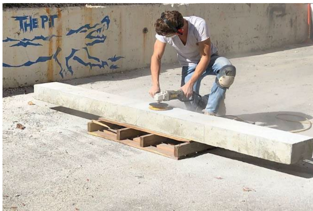
Figure 4-10. Smoothing out imperfections on the leveling pads with a grinder.
