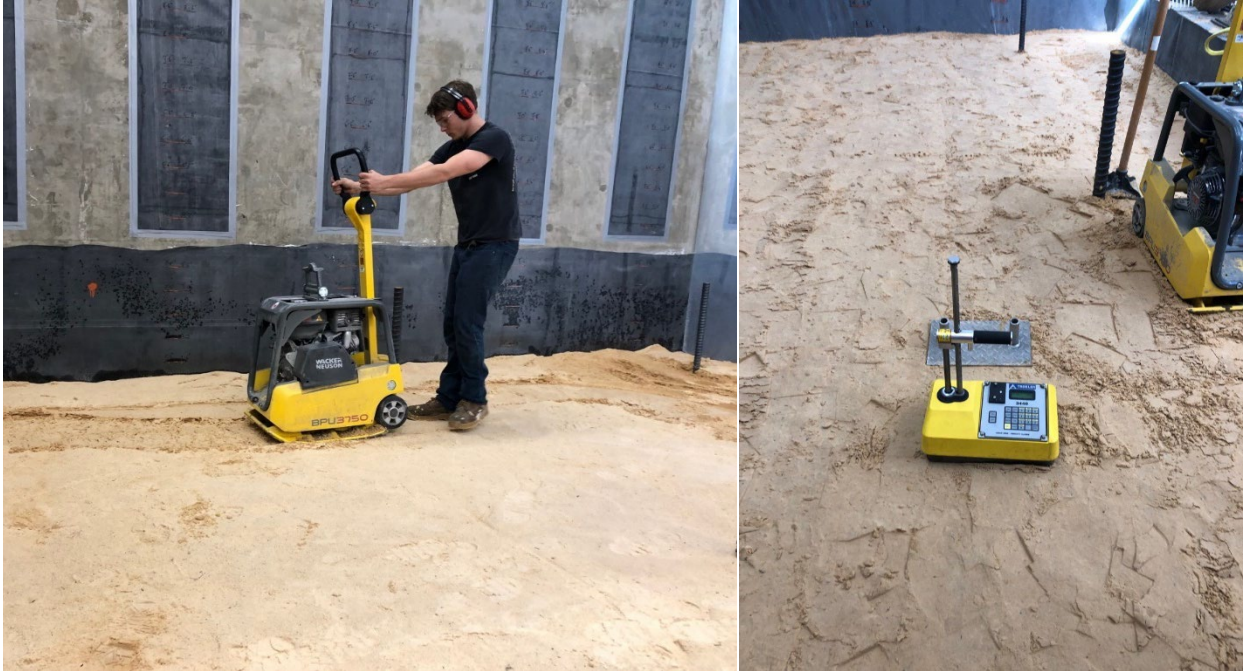
Figure 4-7. Base layer soil compaction and nuclear density testing.
