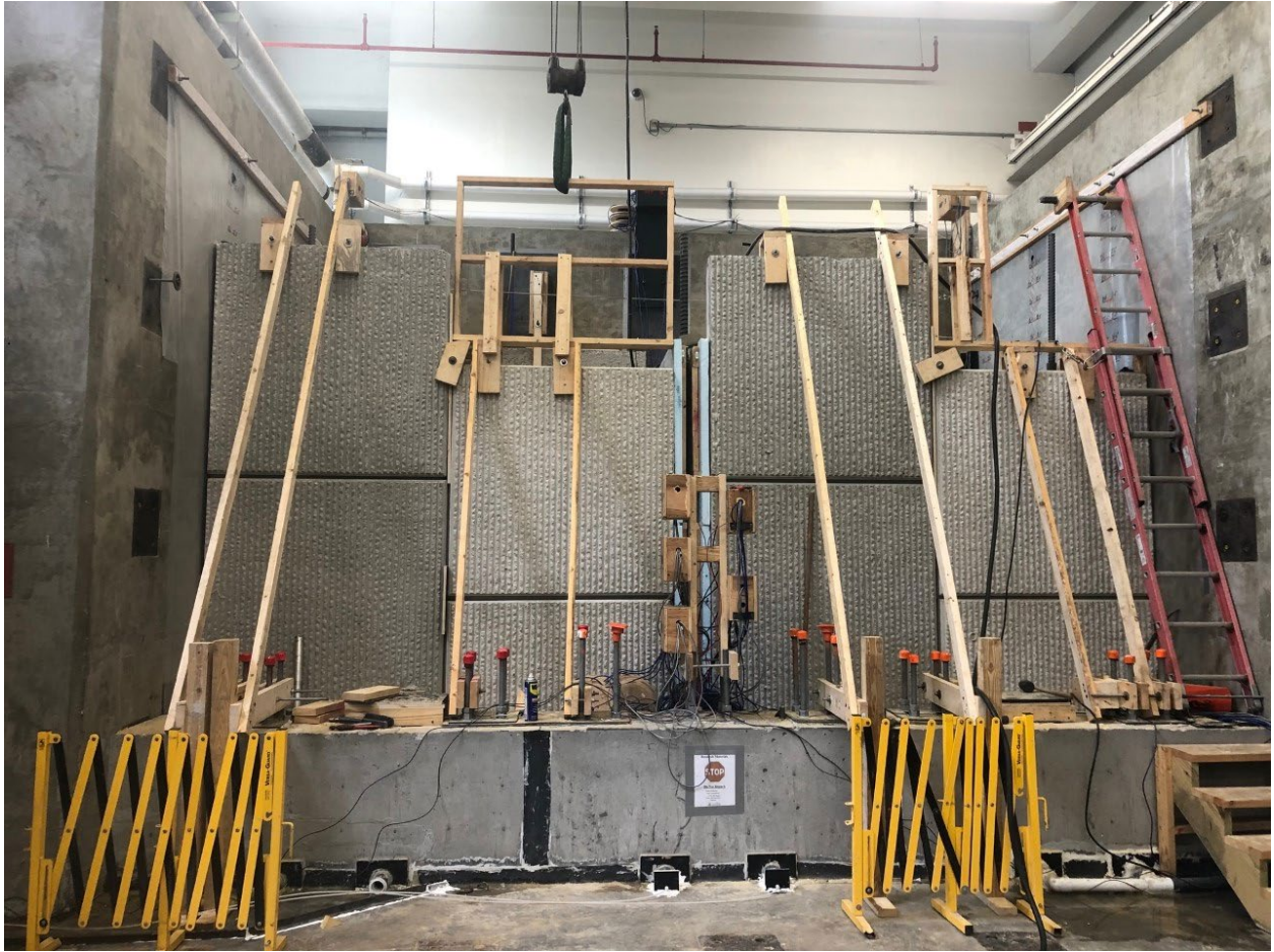
Figure 4-30. Adding the third course of MSE wall panels.
