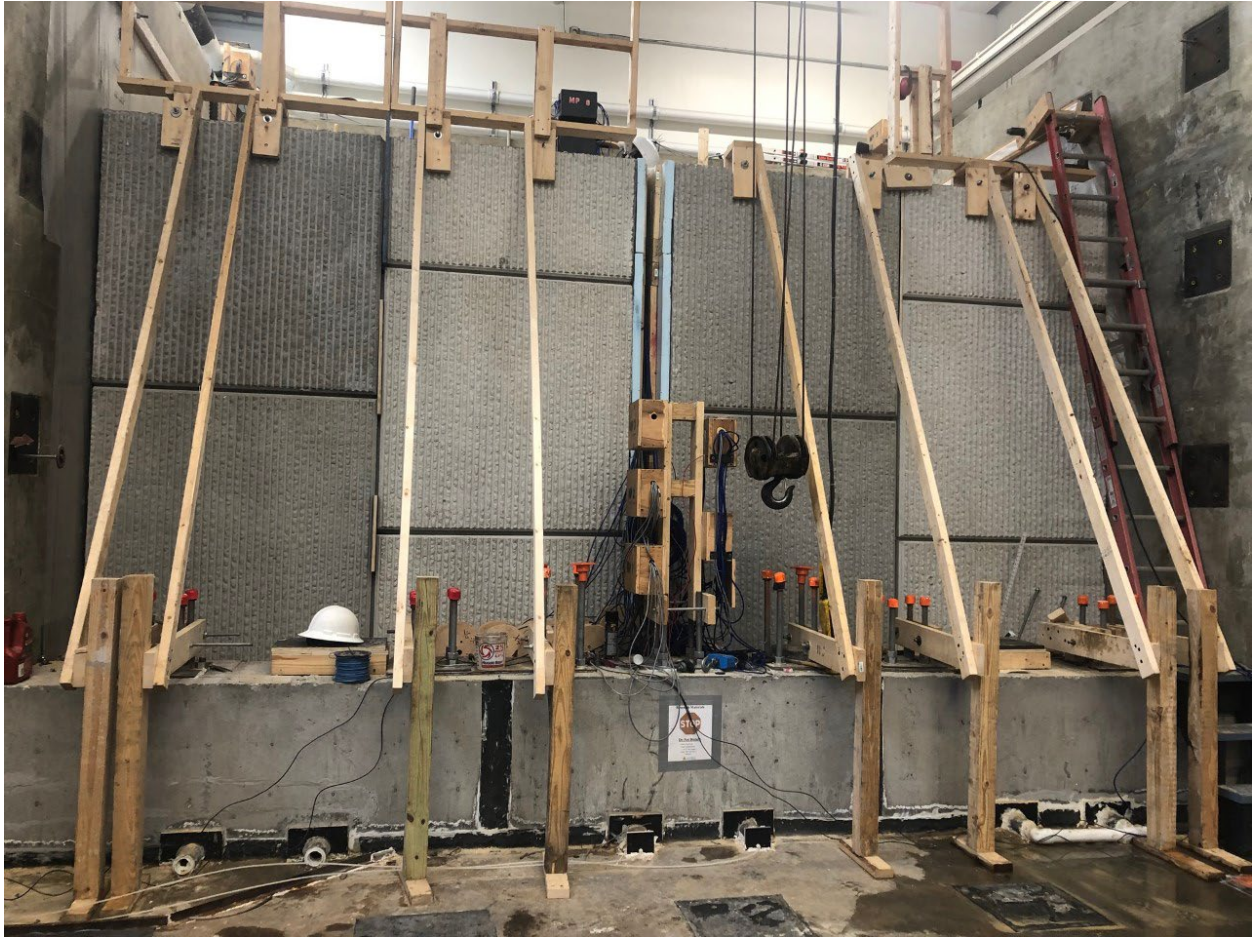
Figure 4-31. Adding the final course of MSE wall panels.
