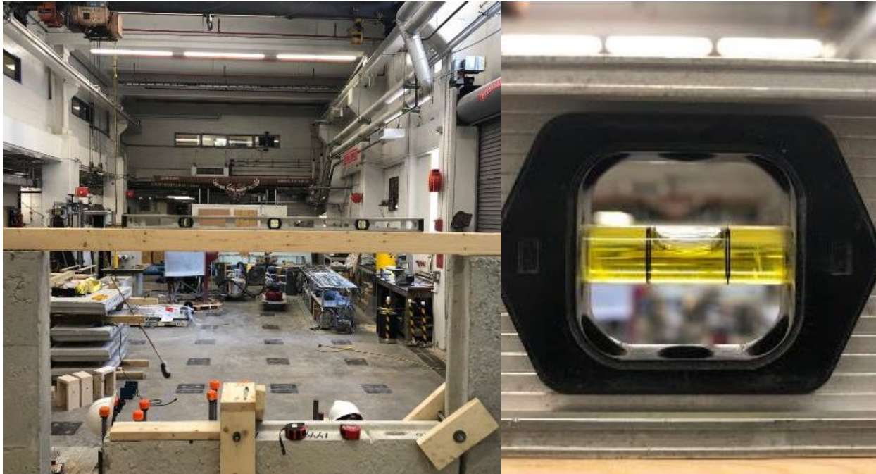
Figure 4-15. Checking the level of frontside MSE panels between the two compaction sides.
