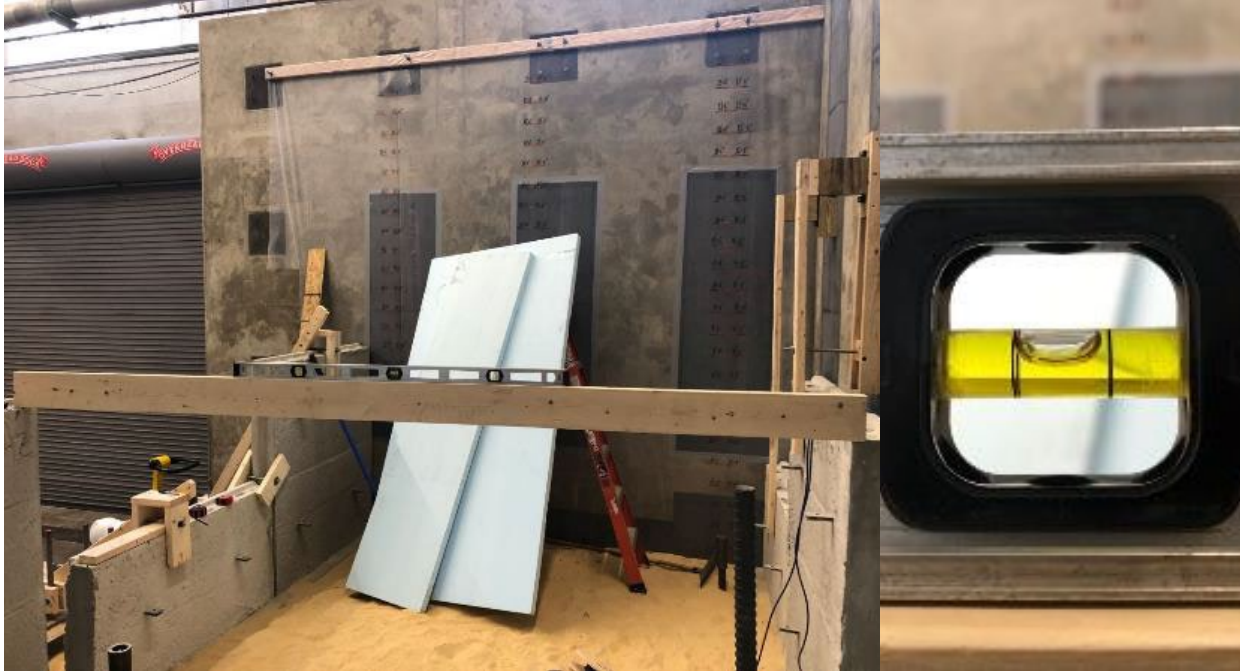
Figure 4-16. Checking the level of the front and back MSE panels.
