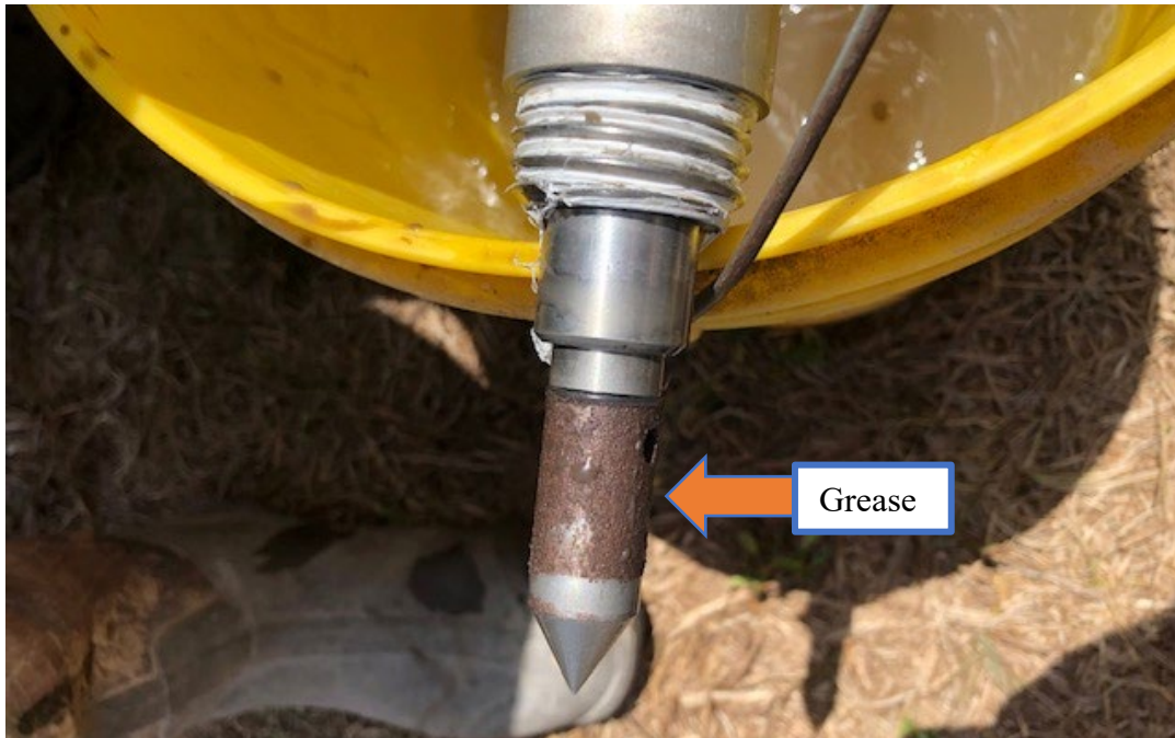
Figure 5-26. Grease transmitted through the drill string and out of the probe.
