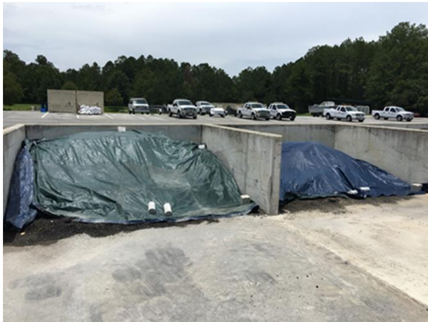
Figure 5-2. Stockpile of RAP covered by plastic sheets
