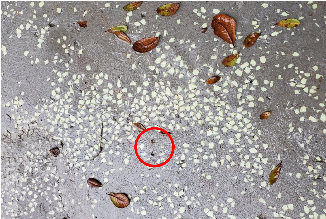
Figure 5-37. A zoomed in look at one of the areas where stones were not well integrated.
