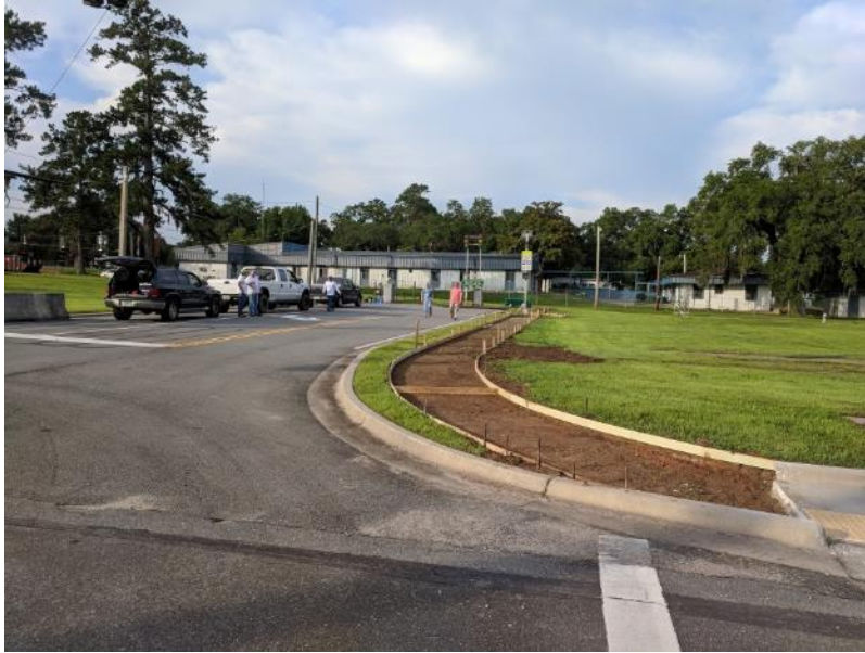
Figure 4-15. Site leveling and preparation for concrete installation
