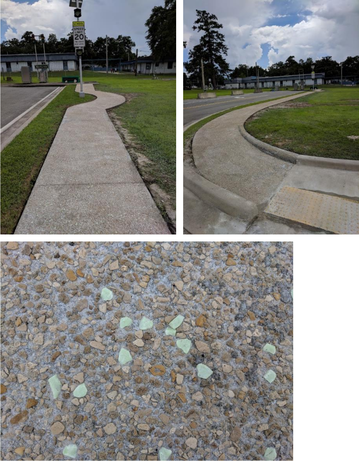
Figure 4-19. Pictures of the final concrete installation (top) and a zoomed-in image showing the exposed surface with glowing stones well integrated (bottom).
