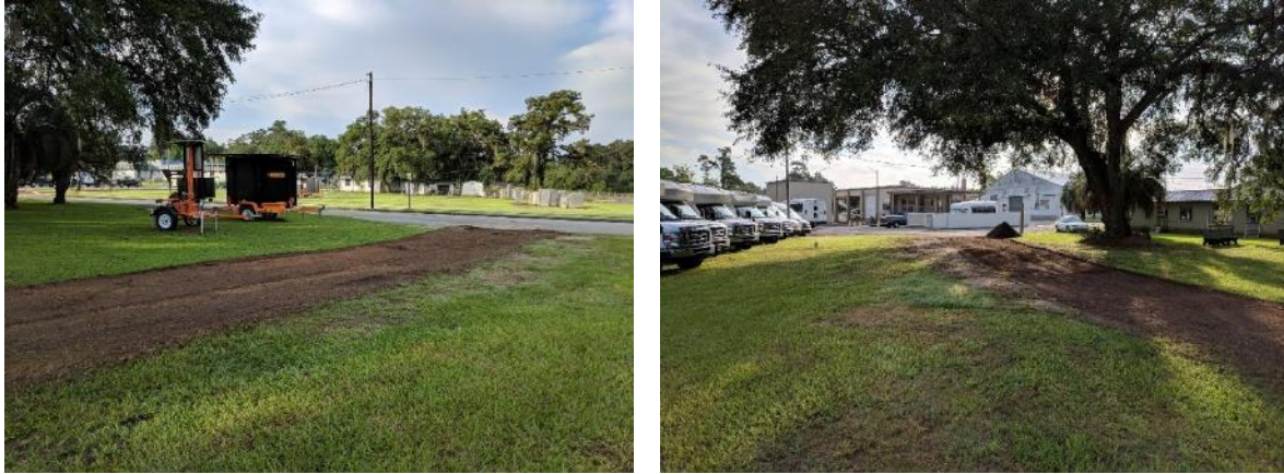
Figure 4-20. Prepped and leveled asphalt site, prior to application.
