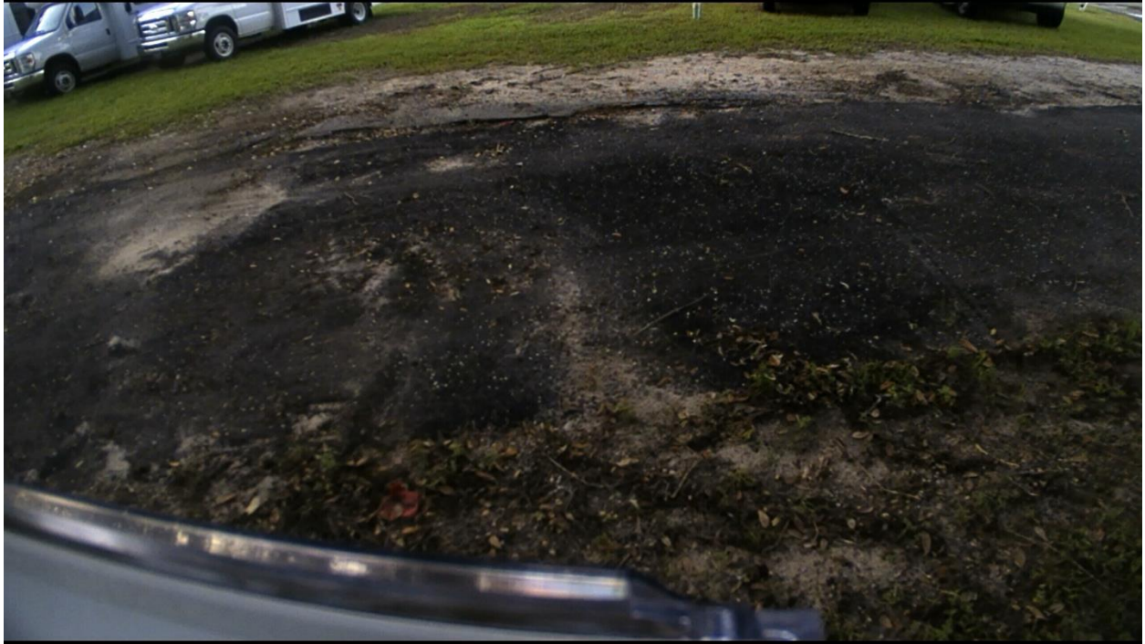
Figure 4-31. Brinno time-lapse photographs of the asphalt installation at 7:00 pm on 10/6/2018.
