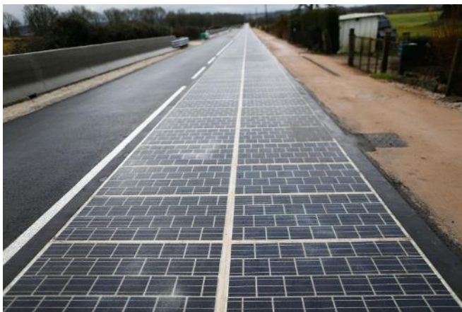
Figure 1-2. Image of a 1-km stretch of solar roadway surface in Normandy, France, completed using Colas’s solar modules 4 .
