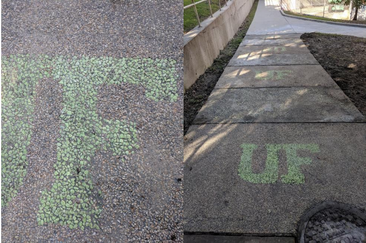
Figure 5-7. Left) Zoomed-in image of the logo after removing the top layer of concrete. Right) Image of the entire installation showing alternating logos and high density stones.
