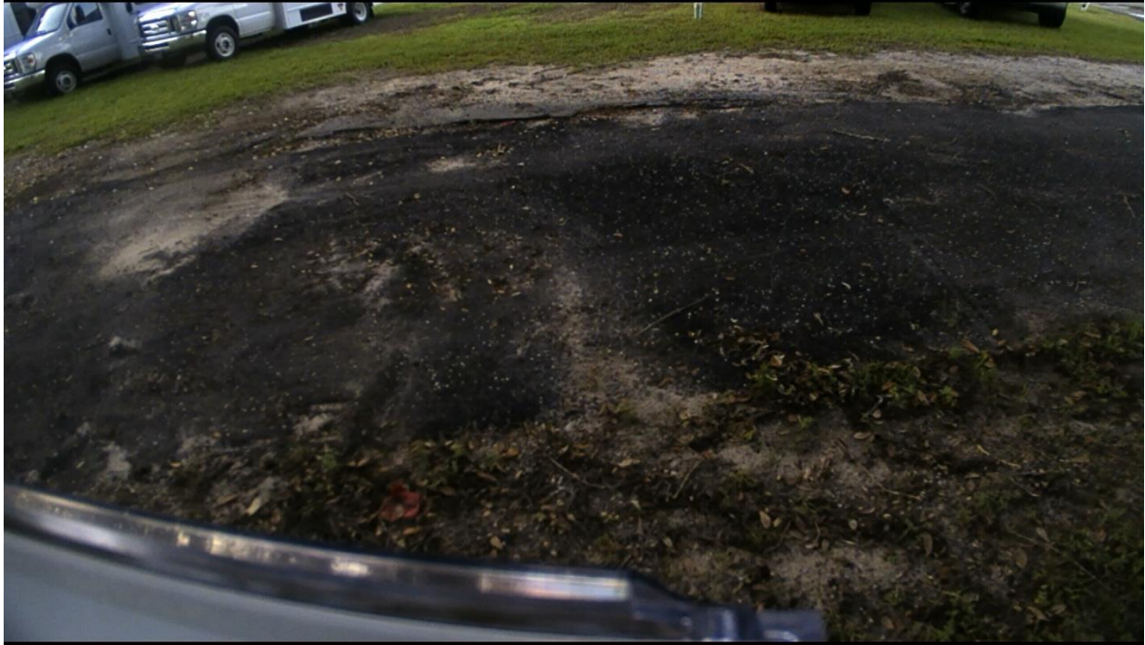
Figure 4-31. Brinno time-lapse photographs of the asphalt installation at 7:00 pm on 10/6/2018.
