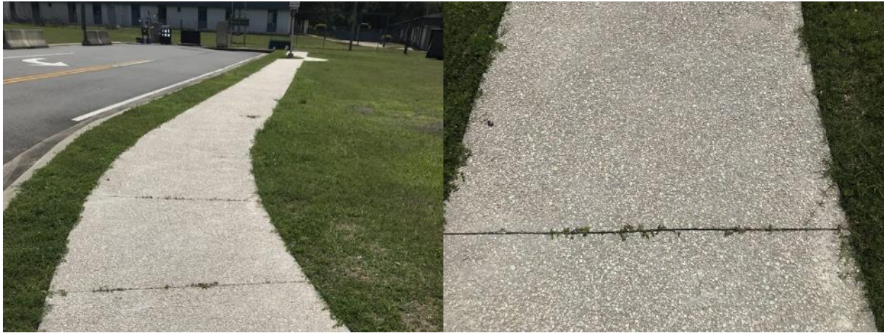
Figure 4-44. Zoomed-out images of the concrete walkway. At this scale, the stones are not easily discernable. Weeds have grown in along the edges of the concrete and within the saw cuts, but there is no noticeable deterioration of the installation.
