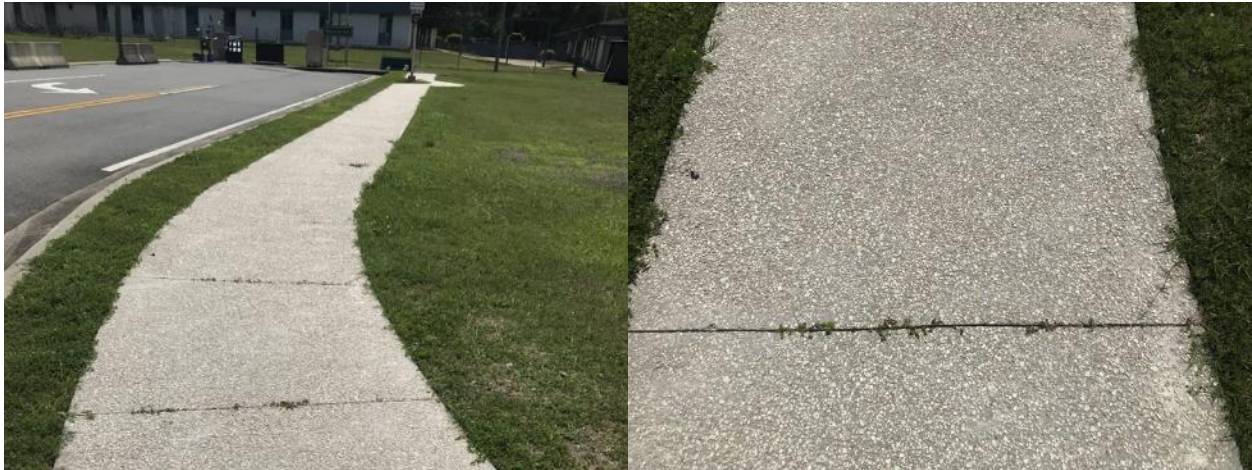
Figure 4-44. Zoomed-out images of the concrete walkway. At this scale, the stones are not easily discernable. Weeds have grown in along the edges of the concrete and within the saw cuts, but there is no noticeable deterioration of the installation.
