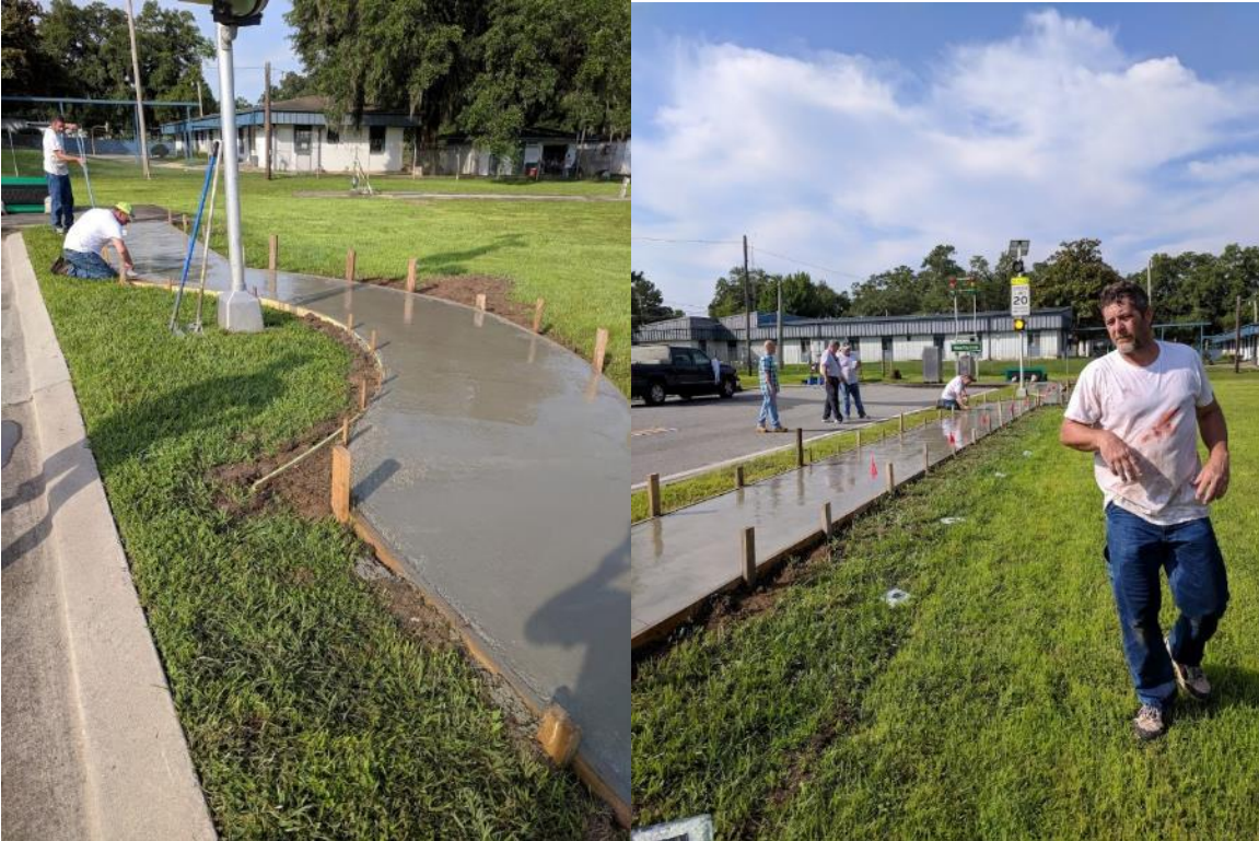
Figure 4-16. Concrete installation immediately following concrete pour and smoothing
