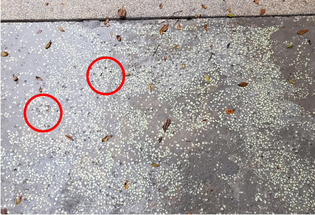
Figure 5-36. In this section of the installation, prefabricated sheets were used and then everything was sanded and ground down to make the surface smooth. In general, the glowing stones are all well integrated, but some were removed after the back covering was peeled away. Selected sections where stones are removed are indicated with the red circles.
