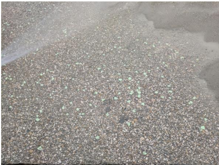
Figure 4-18. Top surface is washed away after 5 hours, revealing the exposed surface and glowing stones.
