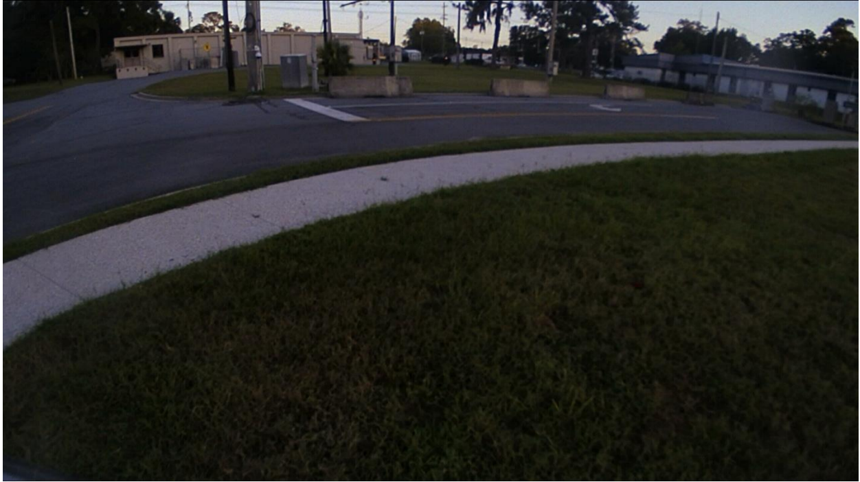
Figure 4-29. Brinno time-lapse photograph of the concrete installation at 7 pm on 10/6/2018.
