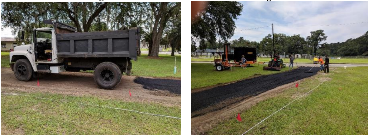
Figure 4-21. Truck used to transport and unload asphalt (left) and smoothing of asphalt by hand after unloading from the truck (right).
