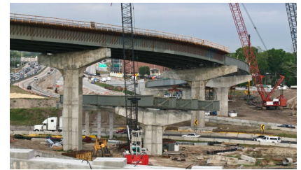
An increasing demand for concrete requires new materials and formulas.
