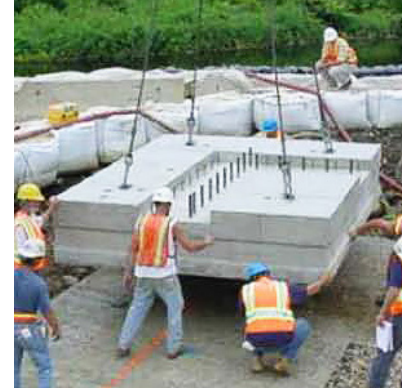
Workers assist as a precast bridge footing is prepared for placement.
