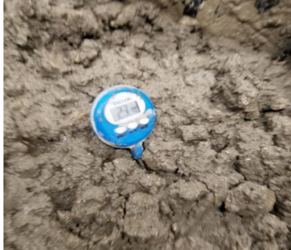
Figure 5-4: Concrete temperature measurement
