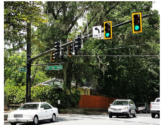
Residual mast arm system capacity allows for the addition of reflective backplates and signs to existing mast arm structures.
