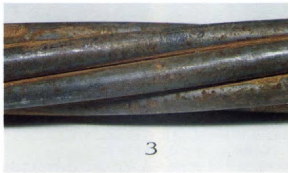
Photo 3. Strand surface before cleaning.
