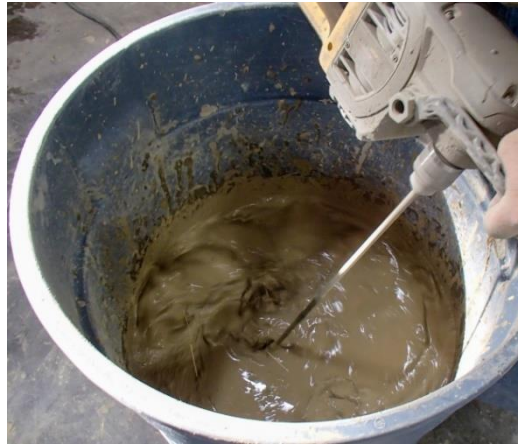
Figure 6-5. Preparation of grout mixture
