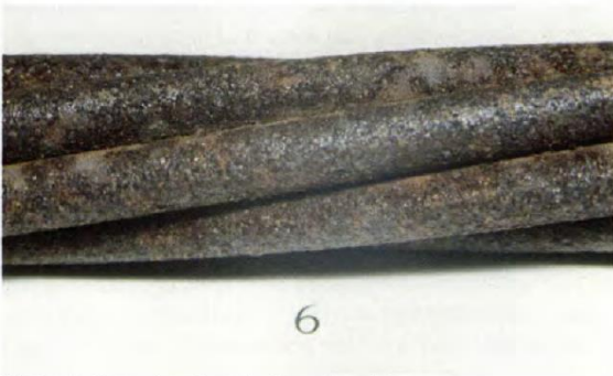
Photo 6. Strand surface before cleaning.
