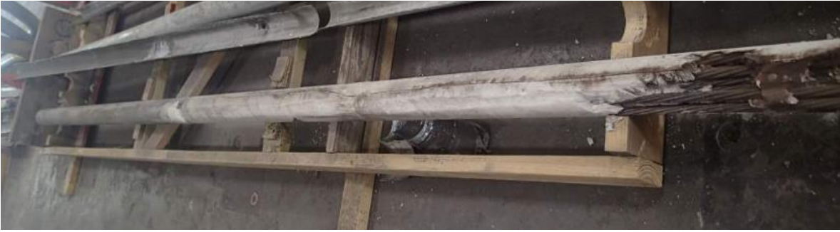
Figure A.3-16. EMT3 after hydrodemolition
