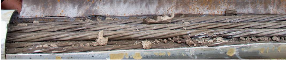
Figure A.4-11. Visual inspection of section 6 after water-blasting
