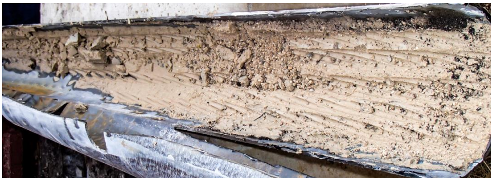
Figure A.4-13. Consistency of remaining grout below strands
