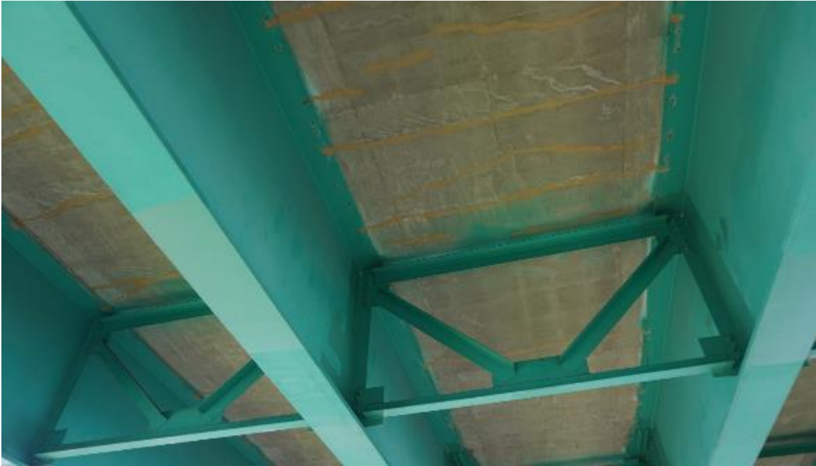
Figure A2-50. 720690 – Typical view of diaphragm between steel girders
