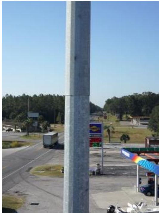
Figure A2-13. 32P054 - View of Lower Slip Joint from Northeast
