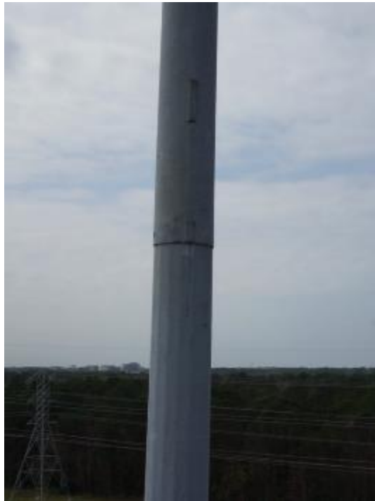
Figure A2-45. 72P743 - View of Second Slip Joint from East
