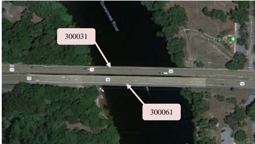
Figure 4-11. Aerial view of 300031 and 300061
