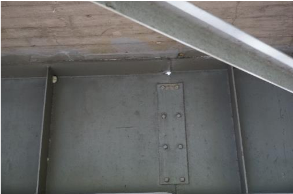
Figure A2-83. 320061 – Typical view of girder splice connection
