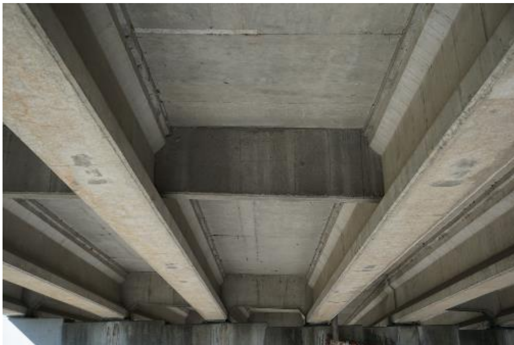
Figure A2-102. 720114 – Typical view down bay between prestressed concrete girders
