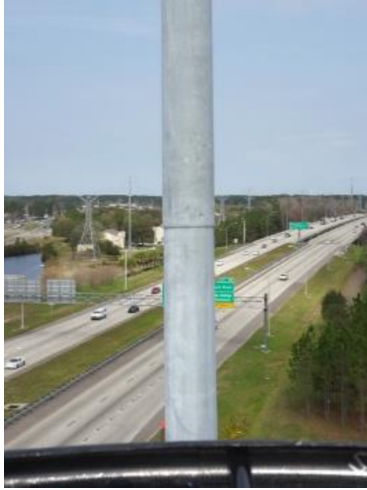
Figure A2-46. 72P743 - View of Second Slip Joint from South
