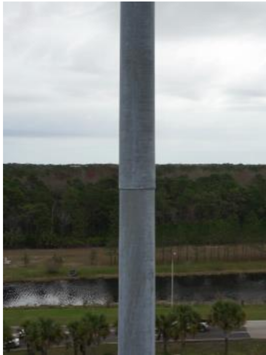
Figure A2-27. 72P740 - View of Second Slip Joint from West
