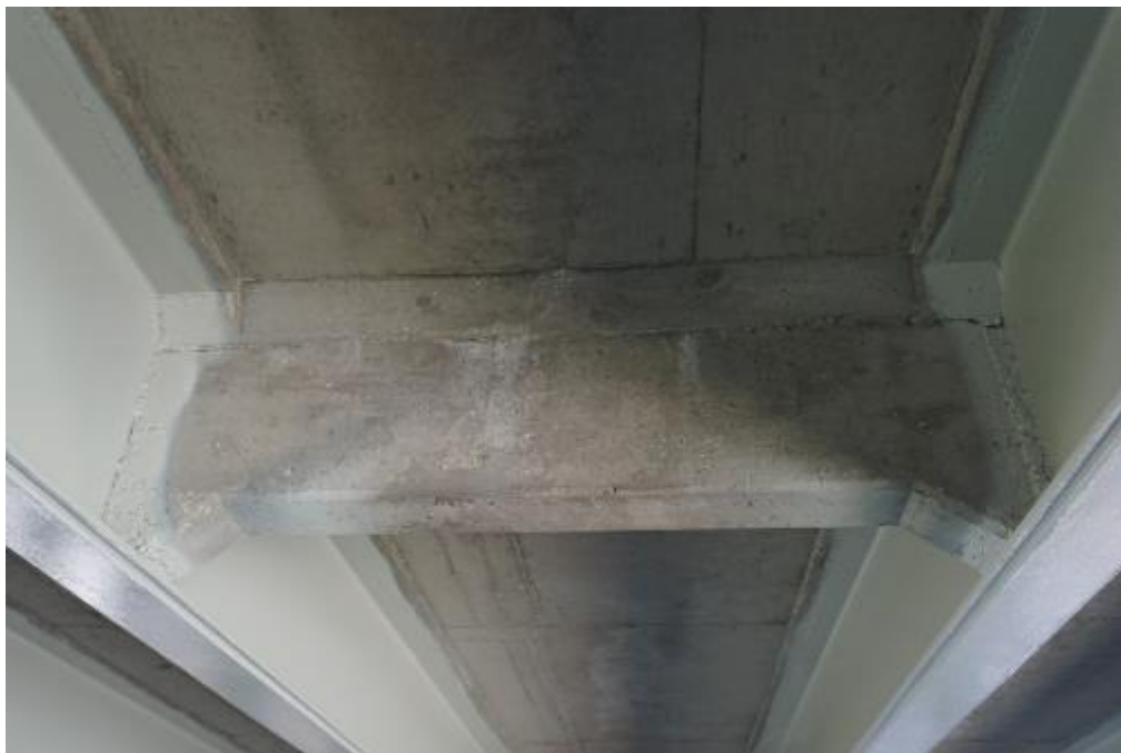
Figure A2-96. 290032 – Typical view of diaphragm between steel beams
