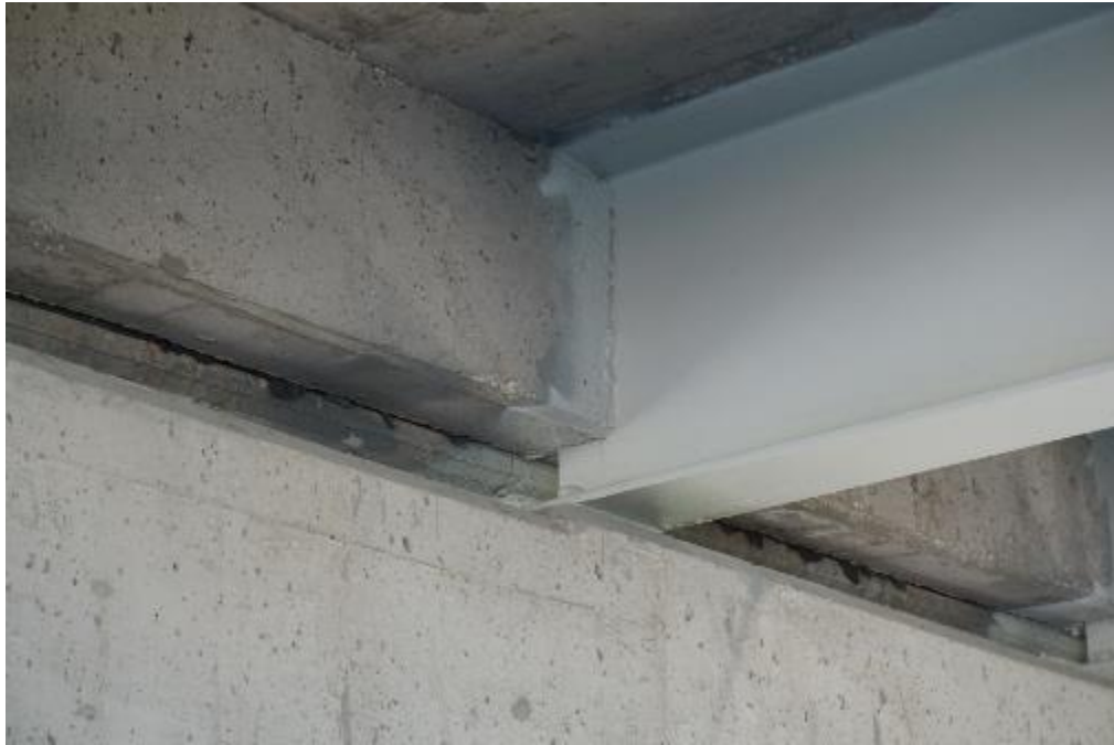
Figure A2-93. 290032 – Typical view of steel beam end
