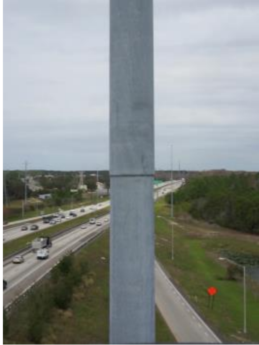
Figure A2-36. 72P741 - View of Second Slip Joint from South
