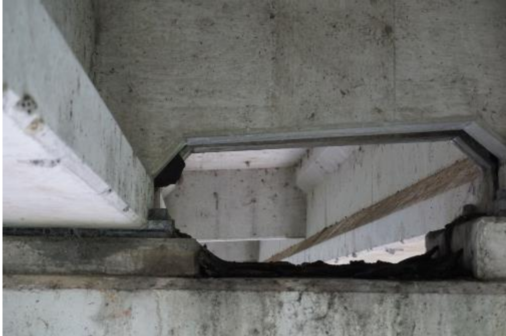
Figure A2-90. 360055 – Typical view of bearing under prestressed concrete girder
