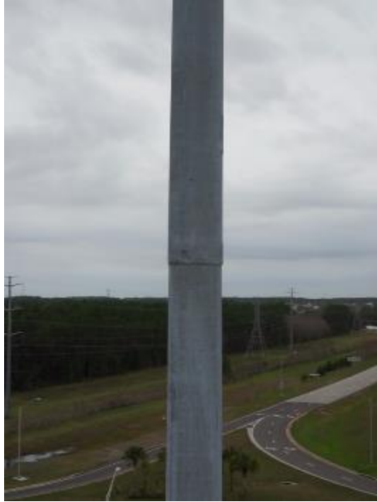
Figure A2-26. 72P740 - View of Second Slip Joint from South
