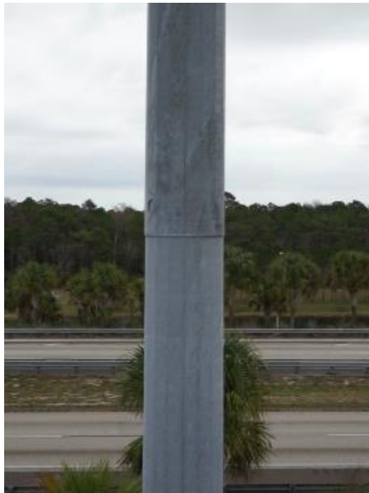
Figure A2-23. 72P740 - View of Lower Slip Joint from West
