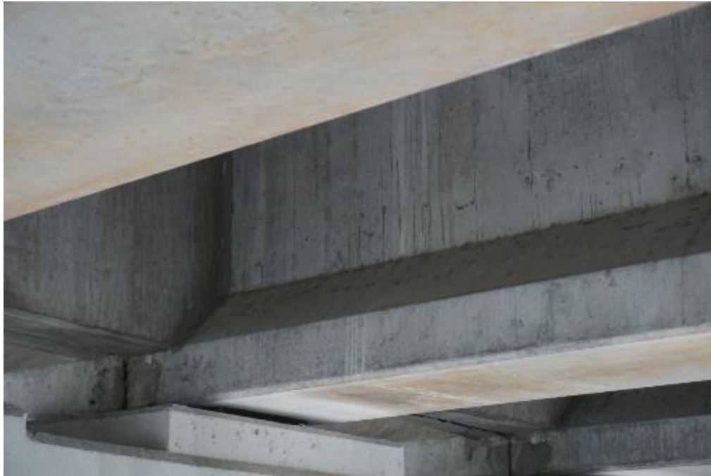
Figure A2-66. 790152 – Typical view of bearing under prestressed concrete girders
