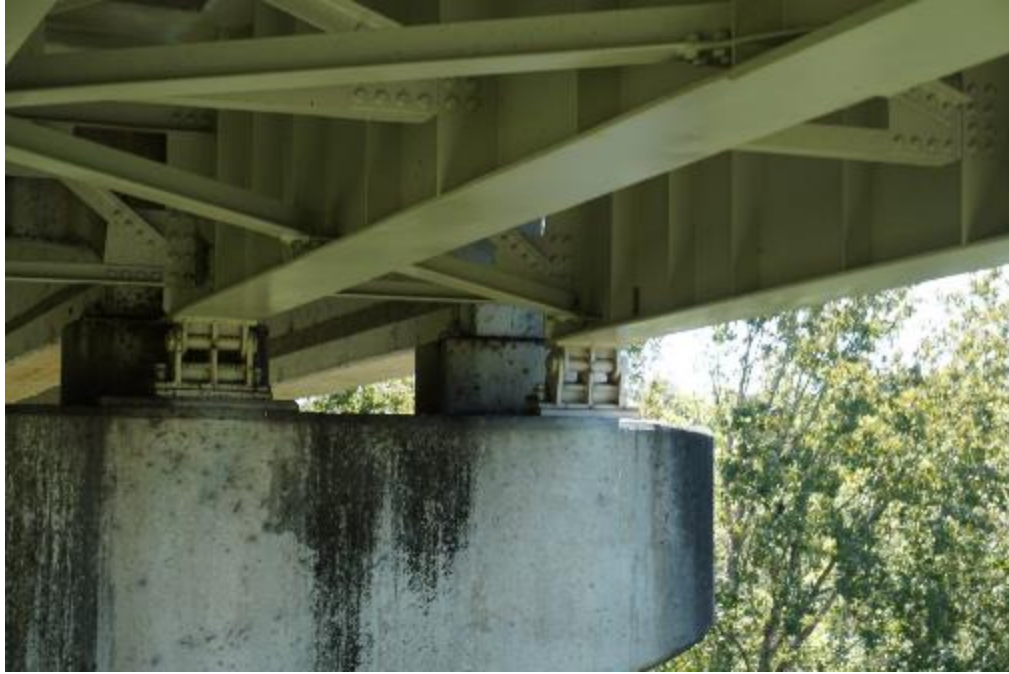
Figure A2-92. 360055 – View of rocker bearing near maximum range of movement
