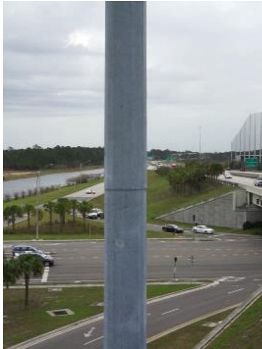
Figure A2-30. 72P741 - View of Lower Slip Joint from North
