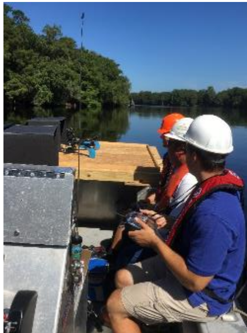
Figure 4-12. Crew, ground station, and sUAV on boat during inspection of 300031 and 300061
