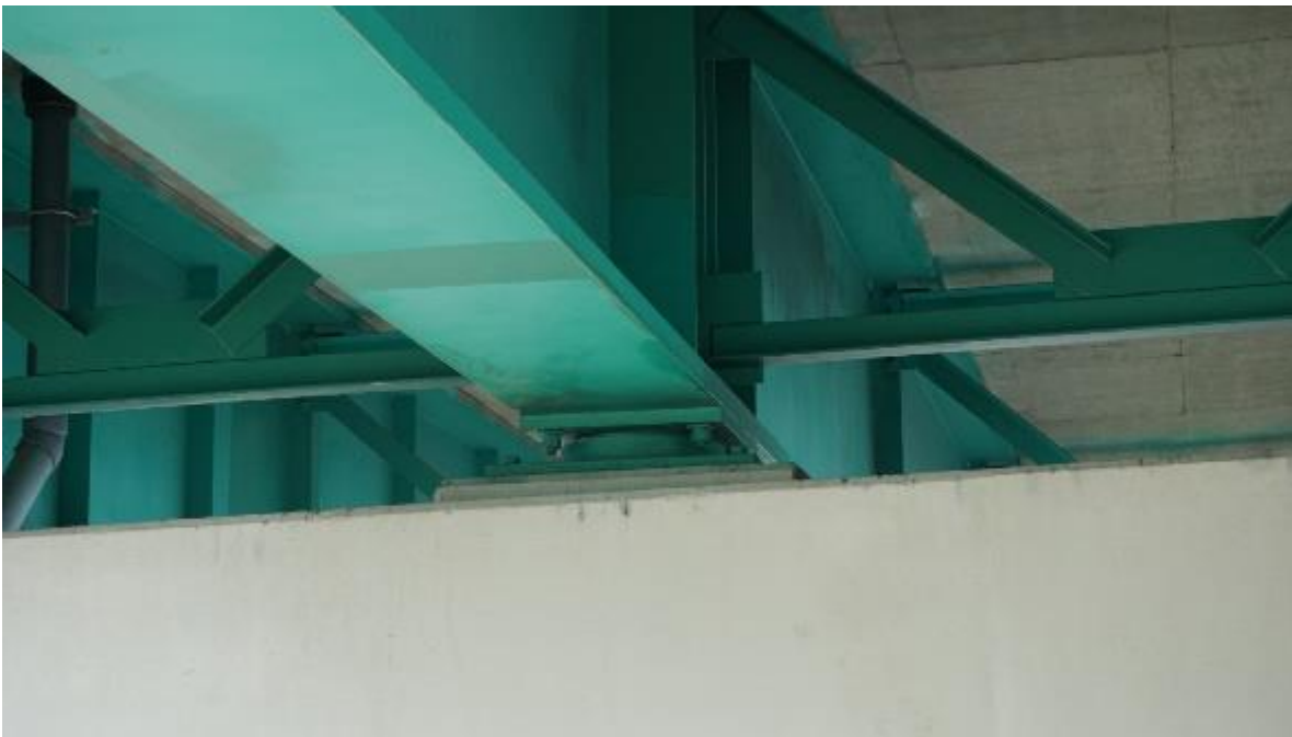
Figure A2-51. 720690 – Typical view of bearing under steel girder
