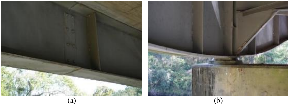
Figure 4-16. Sample images taken during inspection of 320016: (a) splices in the girders, and (b) bearing over Pier Cap 5.
