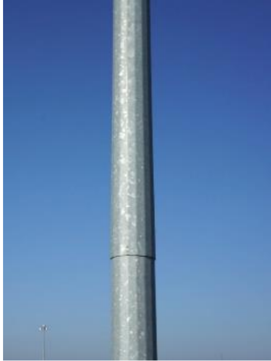
Figure A2-9. 32P050 - View of Second Slip Joint from Southeast
