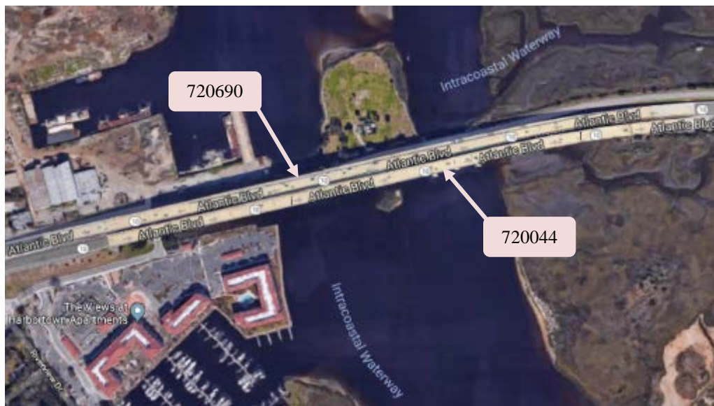
Figure 4-2. Aerial view of 720044 and 7206690
