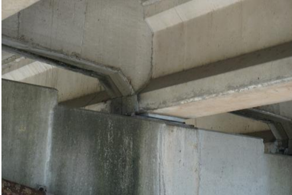
Figure A2-103. 720114 – Typical view of bearing under prestressed concrete girder
