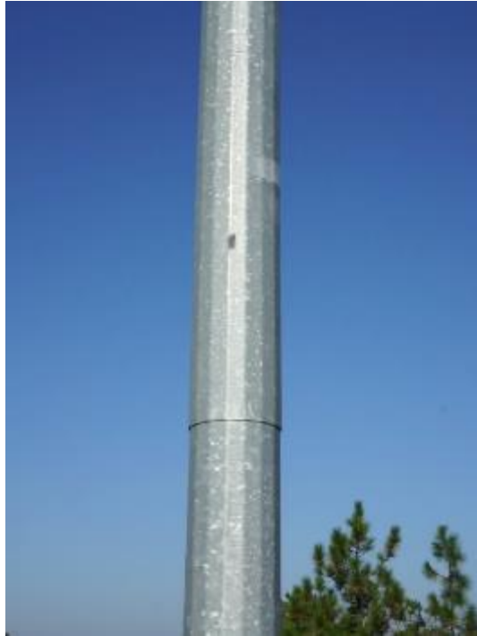
Figure A2-7. 32P050 - View of Lower Slip Joint from Southeast
