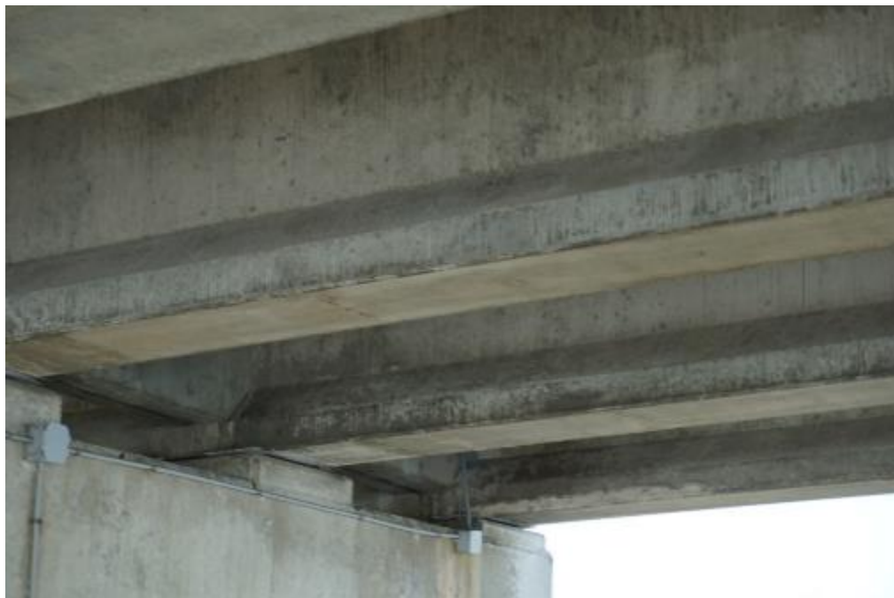
Figure A2-58. 790148 – Typical view of pier cap
