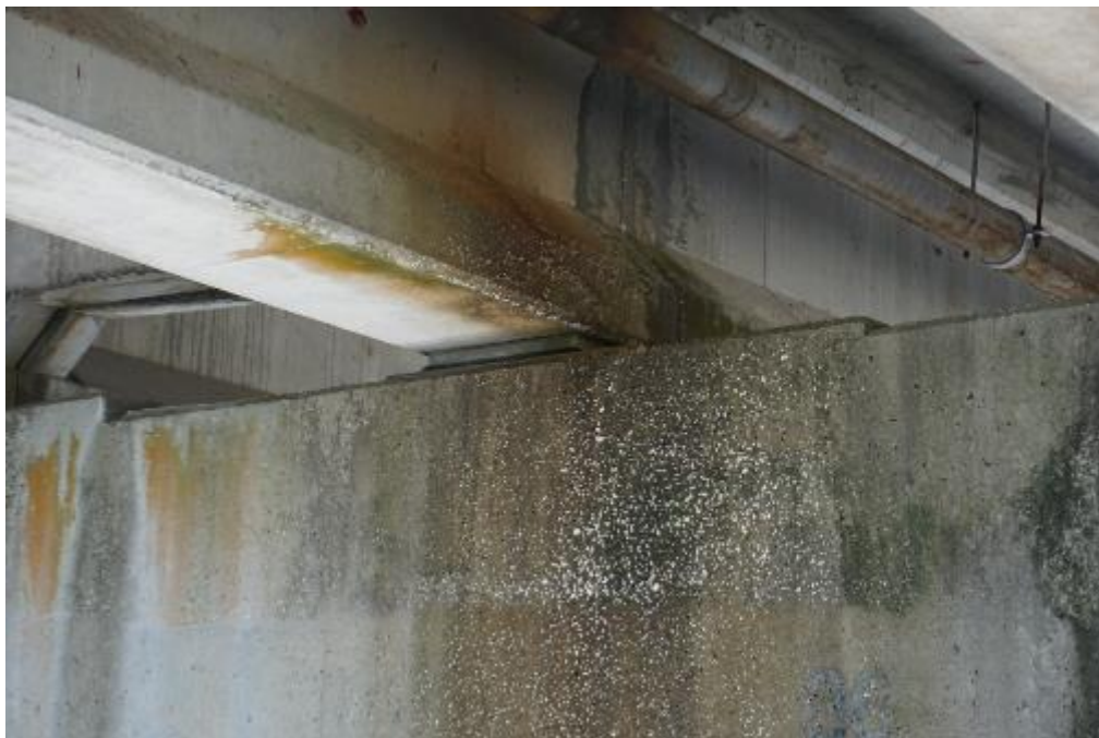
Figure A2-104. 720114 – Typical view of bearing under prestressed concrete girder
