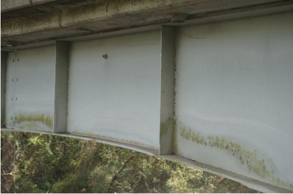
Figure A2-84. 320061 – Typical view of exterior of girder
