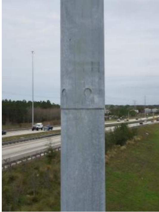
Figure A2-32. 72P741 - View of Lower Slip Joint from South
