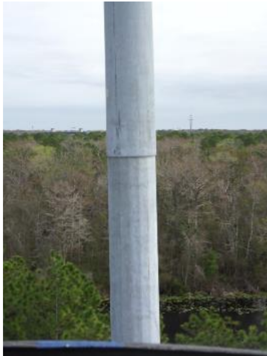
Figure A2-47. 72P743 - View of Second Slip Joint from West
