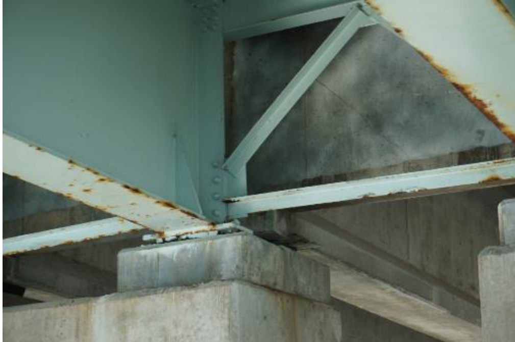
Figure A2-63. 790148 – Typical view of bearing under steel girder
