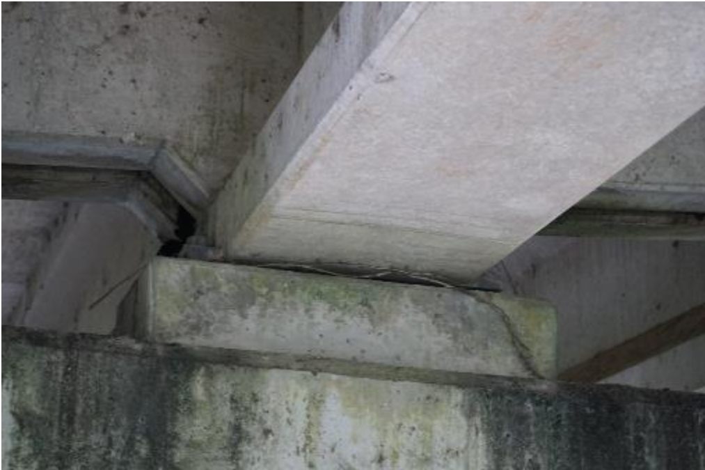
Figure A2-86. 360055 – Typical view of bearing under prestressed concrete girder
