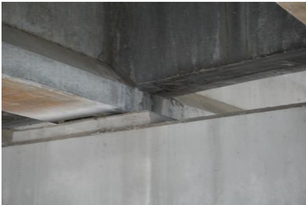
Figure A2-67. 790152 – Typical view of bearing under prestressed concrete girders
