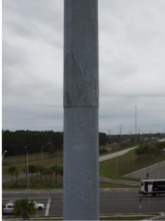
Figure A2-22. 72P740 - View of Lower Slip Joint from South
