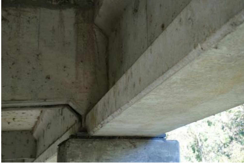
Figure A2-88. 360055 – Typical view of bearing under prestressed concrete girder
