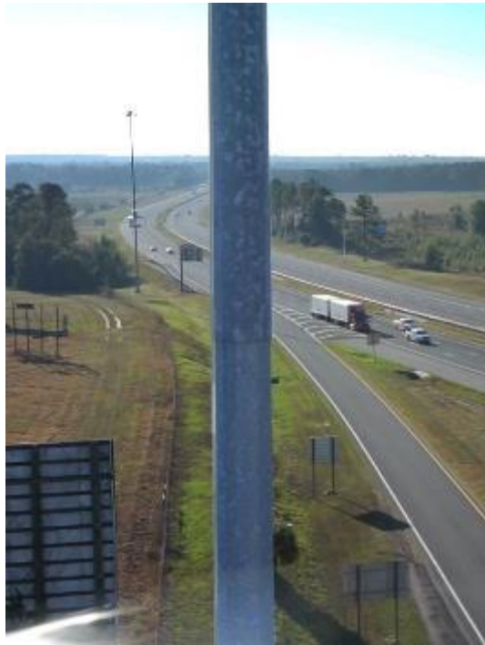
Figure A2-4. 32P049 - View of Second Slip Joint from Northwest
