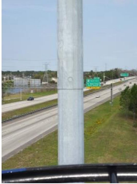
Figure A2-42. 72P743 - View of Lower Slip Joint from South
