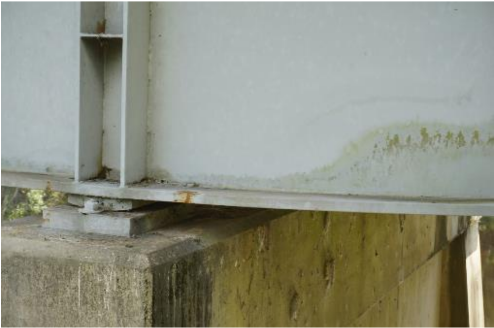
Figure A2-85. 320061 – Typical exterior view of bearing under girder
