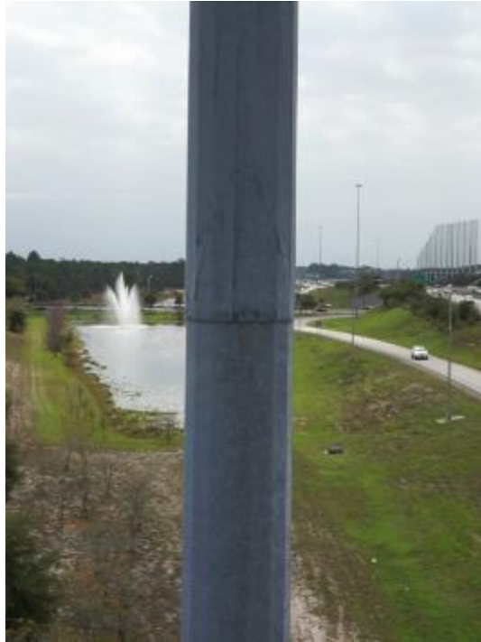
Figure A2-40. 72P743 - View of Lower Slip Joint from North
