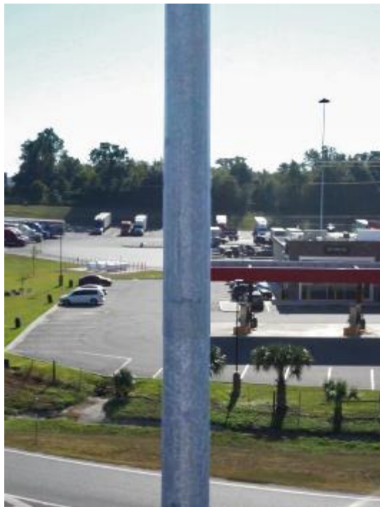
Figure A2-16. 32P054 - View of Lower Slip Joint from Northwest
