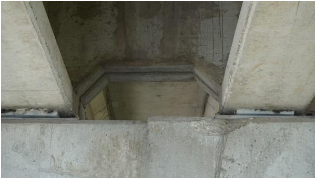
Figure A2-55. 720044 – Typical view of bearing under prestressed concrete girders
