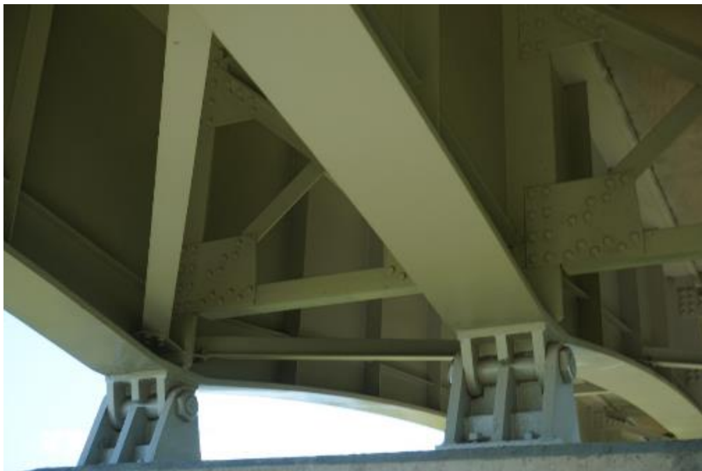
Figure A2-91. 360055 – Typical view of bearing under steel girder
