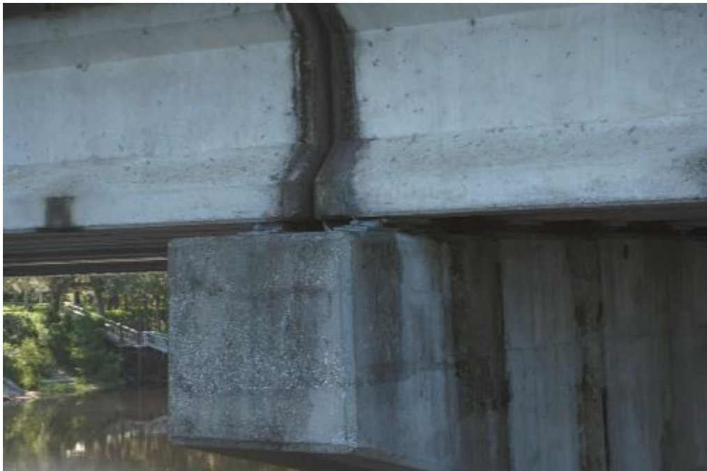
Figure A2-75. 300031 – Typical view of exterior bearings above pier cap
