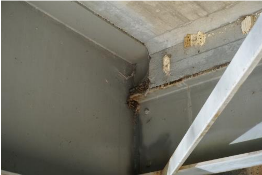
Figure A2-80. 320061 – Typical view of floorbeam connection to girder
