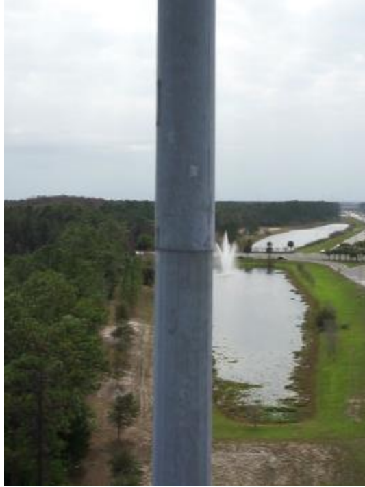
Figure A2-44. 72P743 - View of Second Slip Joint from North
