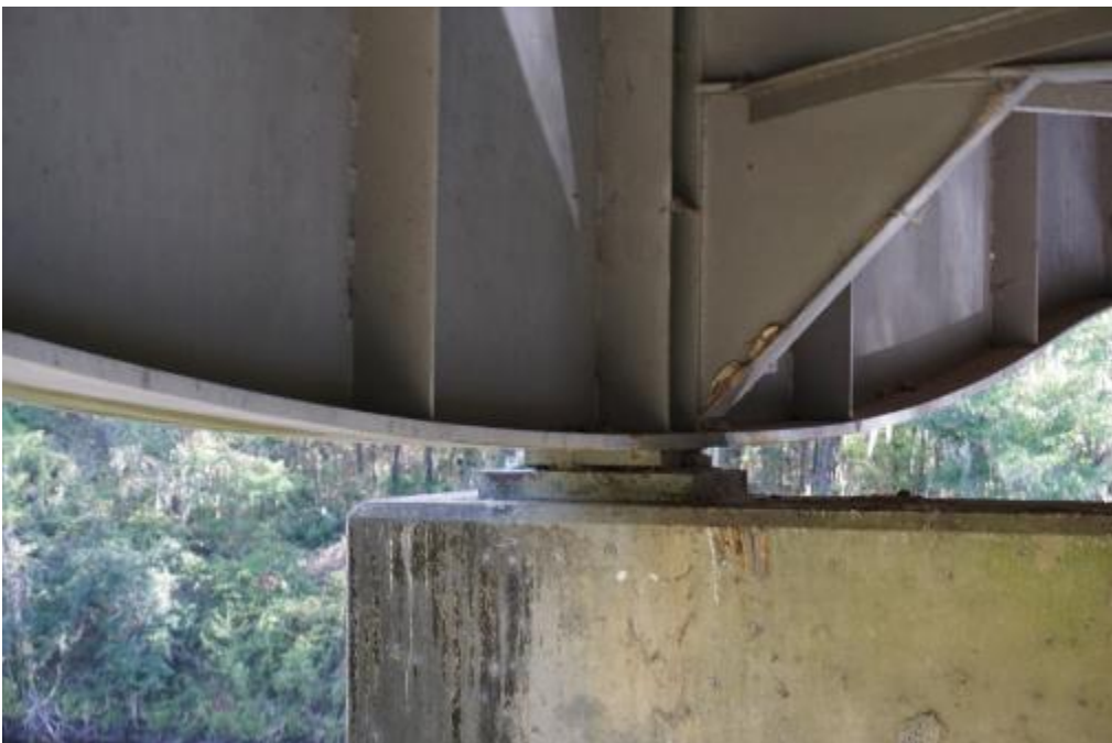
Figure A2-81. 320061 – Typical view of floorbeam connection to girder
