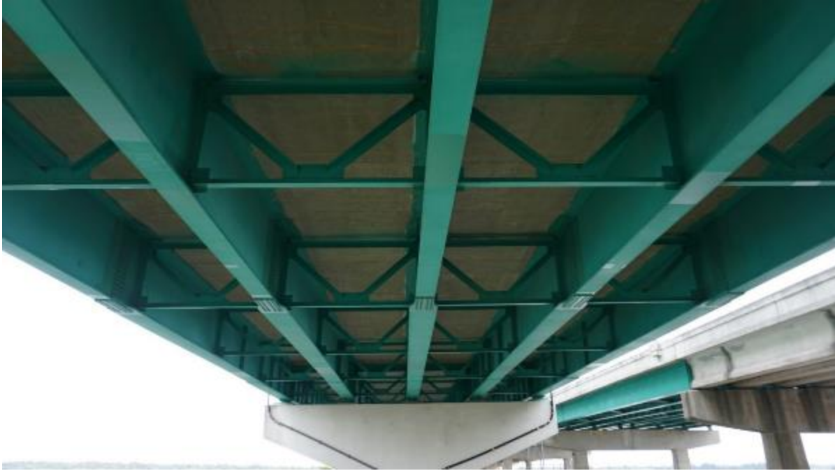
Figure A2-52. 720690 – Typical view down steel girders span
