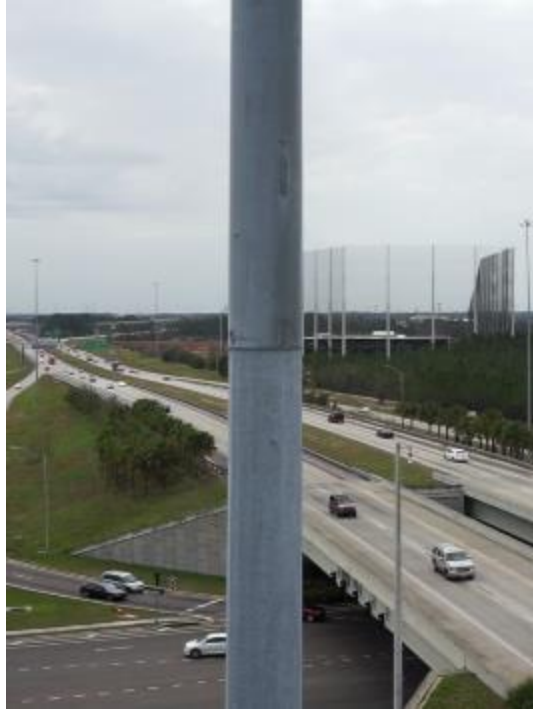
Figure A2-34. 72P741 - View of Second Slip Joint from North
