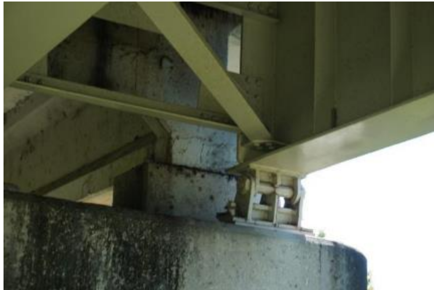
Figure 4-18. Bearing 17-5 over Pier 18
