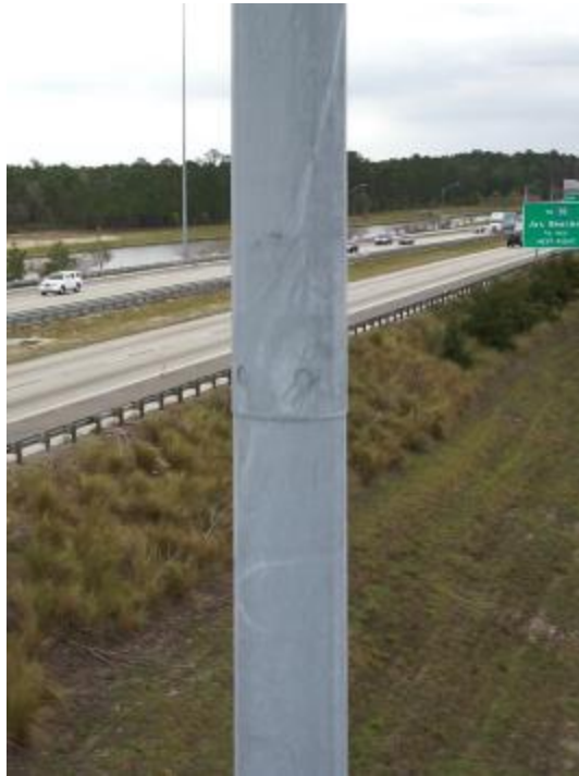
Figure A2-20. 72P740 - View of Lower Slip Joint from North
