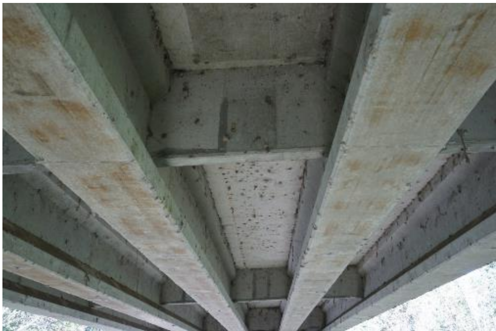
Figure A2-87. 320055 – Typical view down bay between prestressed concrete girders
