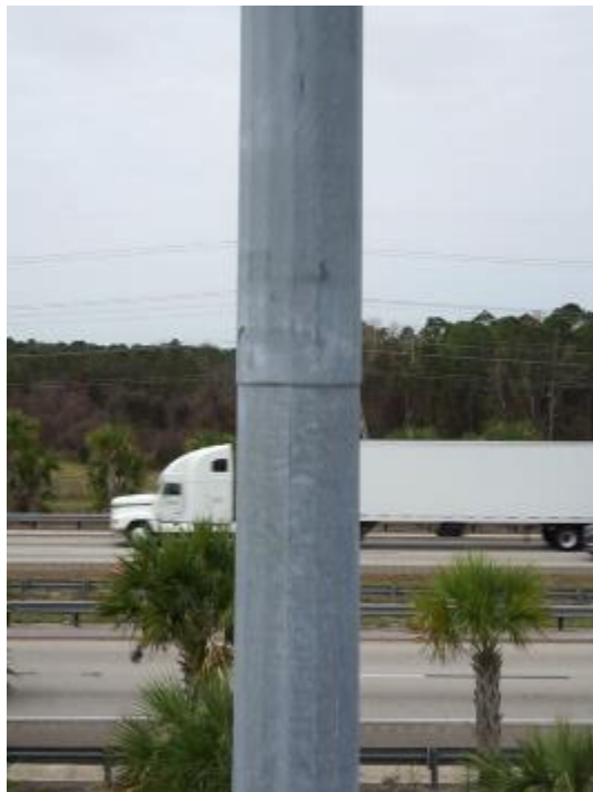
Figure A2-31. 72P741 - View of Lower Slip Joint from East
