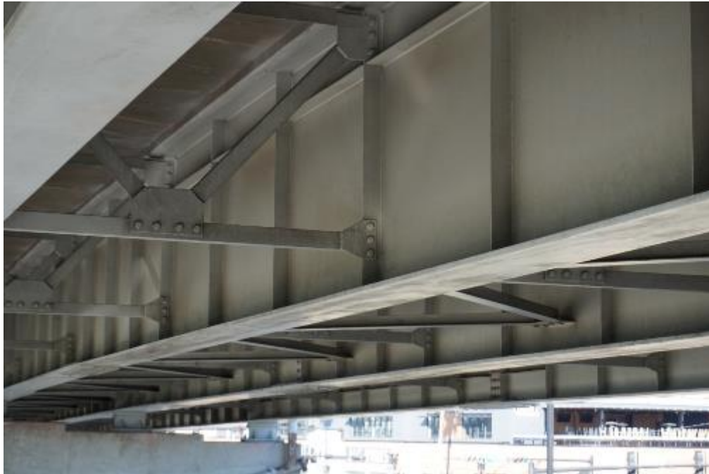
Figure A2-99. 720114 – Typical view of diaphragm between steel girders
