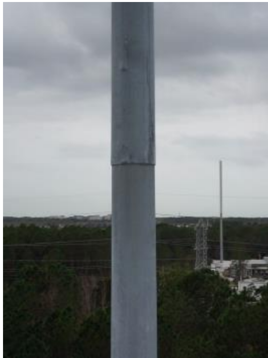
Figure A2-25. 72P740 - View of Second Slip Joint from East
