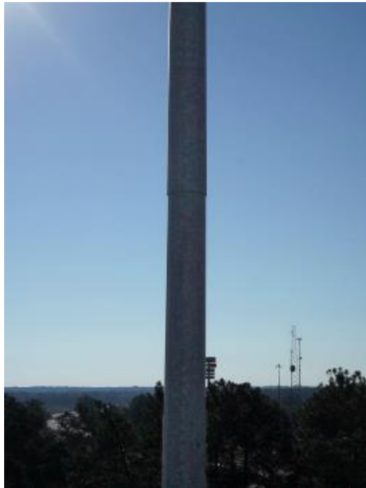
Figure A2-10. 32P050 - View of Second Slip Joint from Northwest
