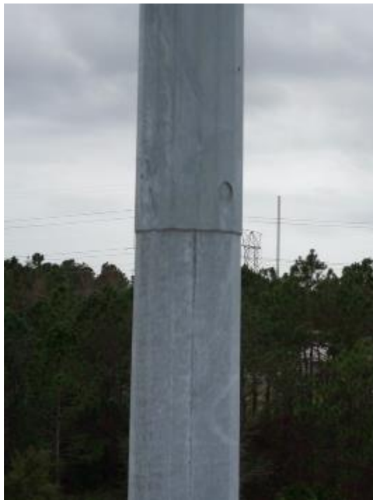
Figure A2-21. 72P740 - View of Lower Slip Joint from East
