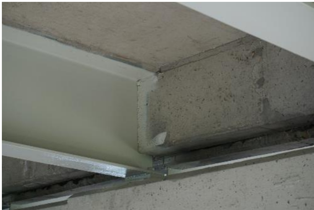
Figure A2-94. 290032 – Typical view of steel beam ends
