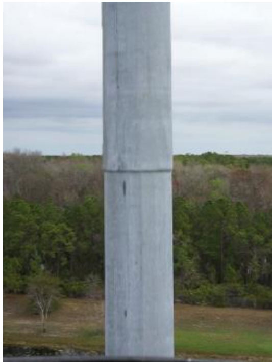
Figure A2-37. 72P741 - View of Second Slip Joint from West
