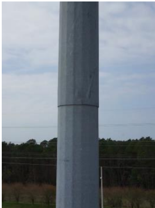
Figure A2-41. 72P743 - View of Lower Slip Joint from East
