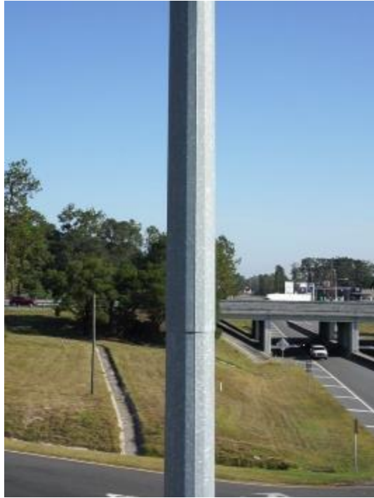
Figure A2-15. 32P054 - View of Lower Slip Joint from Southwest
