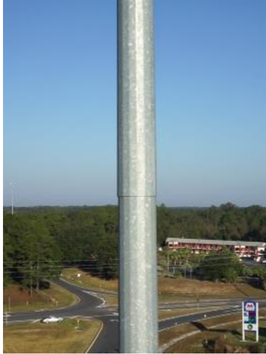
Figure A2-0-3. 32P049 - View of Second Slip Joint from Southeast
