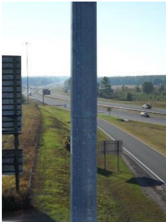
Figure A2-0-2. 32P049 - View of Lower Slip Joint from Northwest
