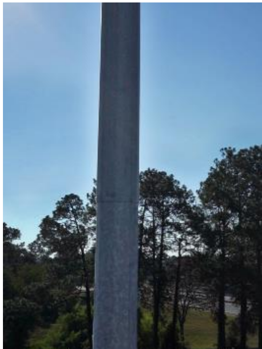
Figure A2-8. 32P050 - View of Lower Slip Joint from Northwest
