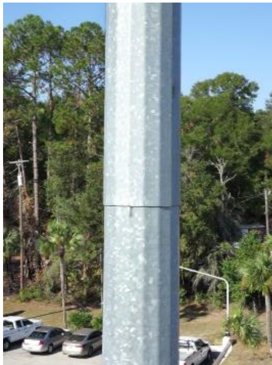
Figure A2-14. 32P054 - View of Lower Slip Joint from Southeast
