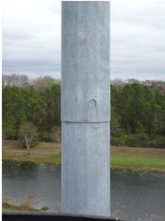
Figure A2-33. 72P741 - View of Lower Slip Joint from West
