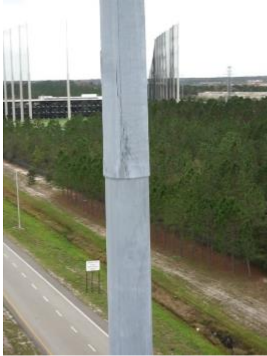
Figure A2-24. 72P740 - View of Second Slip Joint from North
