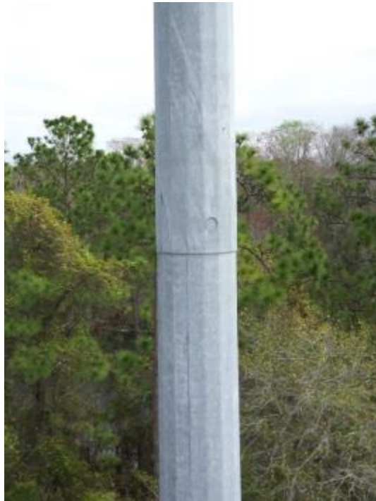
Figure A2-43. 72P743 - View of Lower Slip Joint from West
