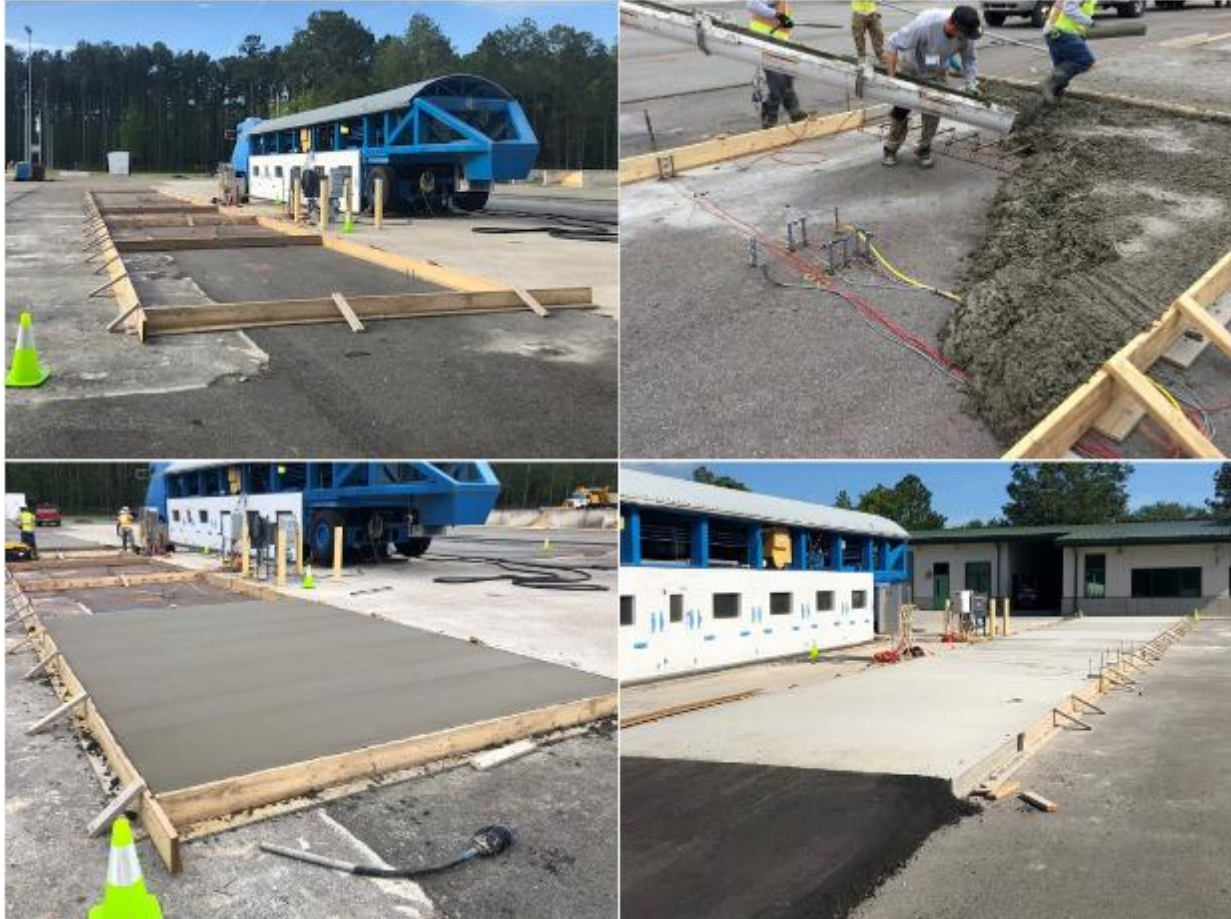
Fig 5.3 Construction of the slabs for Slab Study 2.
