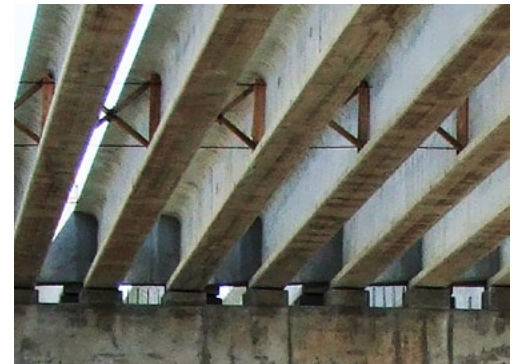
While under construction, bridge girders are cross-braced for stability.
