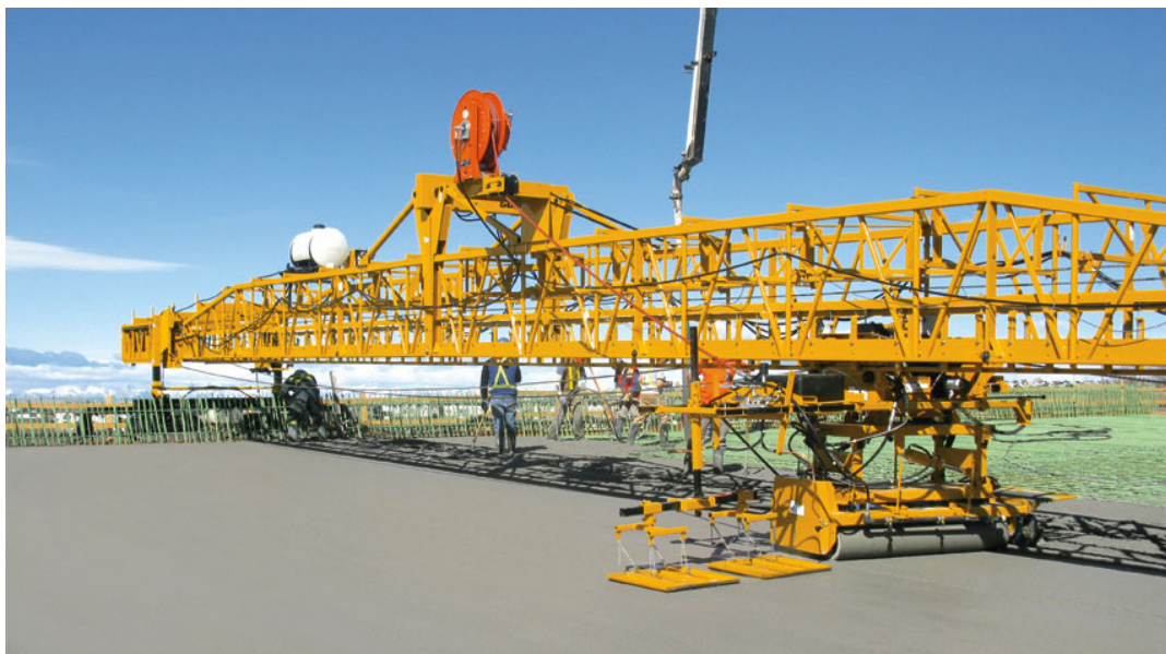
Figure 6.5 Typical bridge deck finishing machine in operation (Photo credit: Gomaco)
