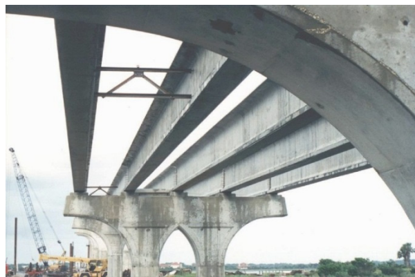
Figure 1.1 Prestressed concrete girders braced together for stability
