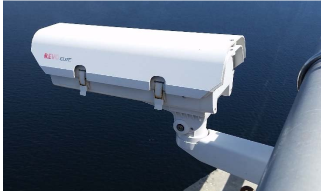
Figure 3-16. Northbound camera on the North Tower.
