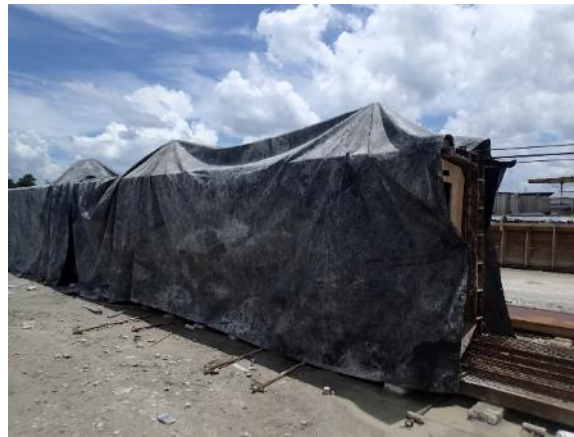
Figure 4-14 Tarp cover used for curing
