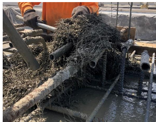
Figure 2-14 Fiber clumping during mixing (Macrosynthetic fiber with length 2.3 in. (58 mm) at volume of 0.7%)
