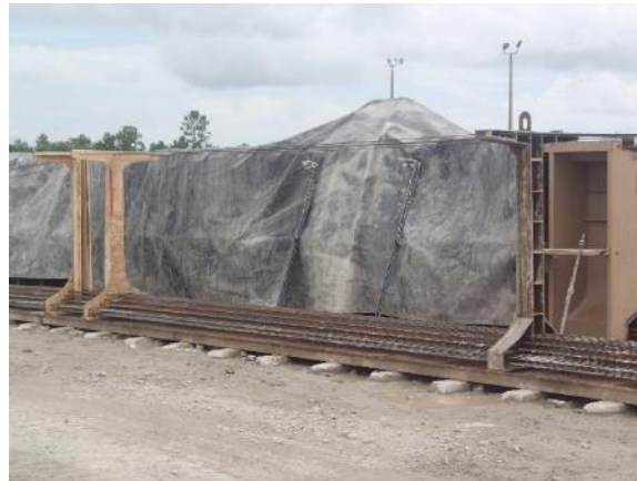
Figure 4-8 Prestressing strands after tension was applied
