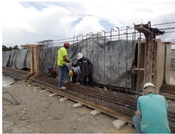
Figure 4-9 Mild steel reinforcement installation
