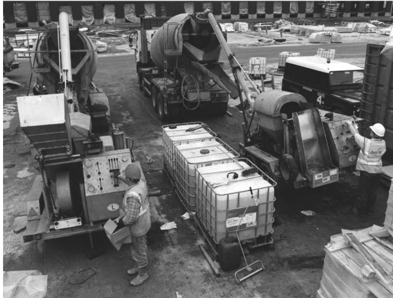
Figure 2-15 Fibers added to truck mixer using fiber blower (ACI 544.3R-08)
