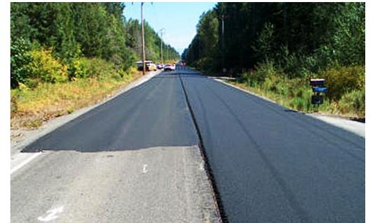
*This photo of a repaving project shows the original road surface (lower left), the interlayer (upper left), and the new pavement surface (right).*
