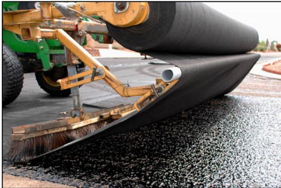
(a) Nonwoven geotextiles
