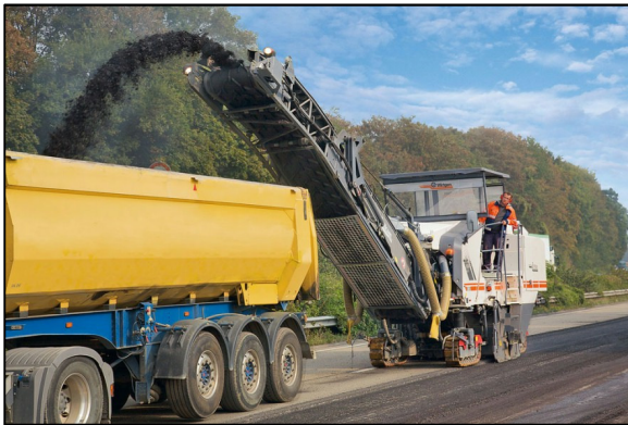
(a) Milling and replacing ( www.wirtgen-group.com )
