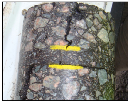
Figure 5-6. Crack jumping phenomenon (Bennert et al., 2011)
