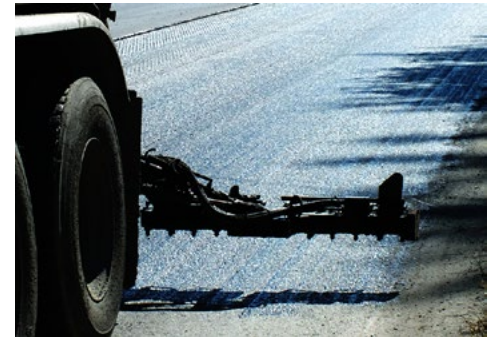
An even layer of tack coat is essential for ensuring good bonding between layers of asphalt.
