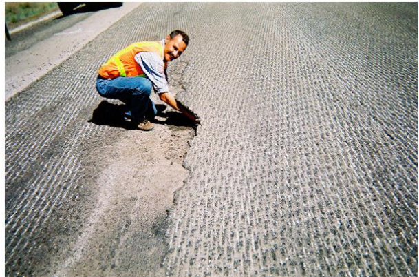
f. Thin debonded layer after milling on SR 97A
