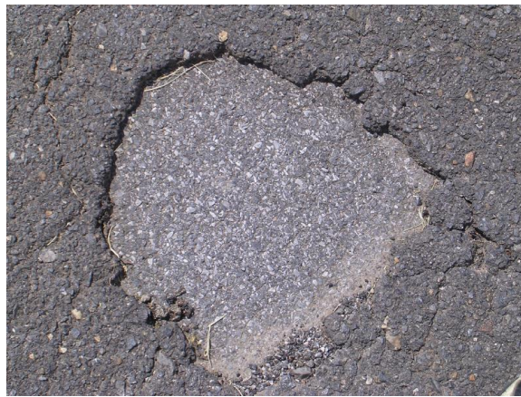
b. Delamination of surface layer
