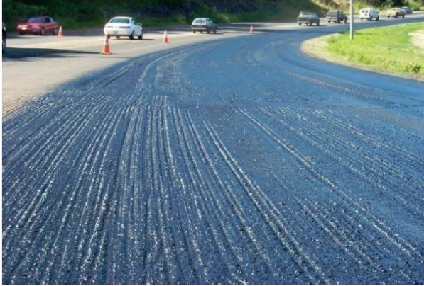
a. Good coverage on SR 101 (milled surface)
