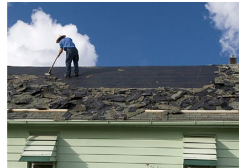
Reroofing generates 10 million tons of asphalt shingle waste each year in the U.S.
