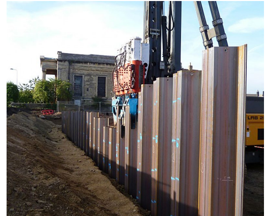
Installation of a sheet wall pile.
