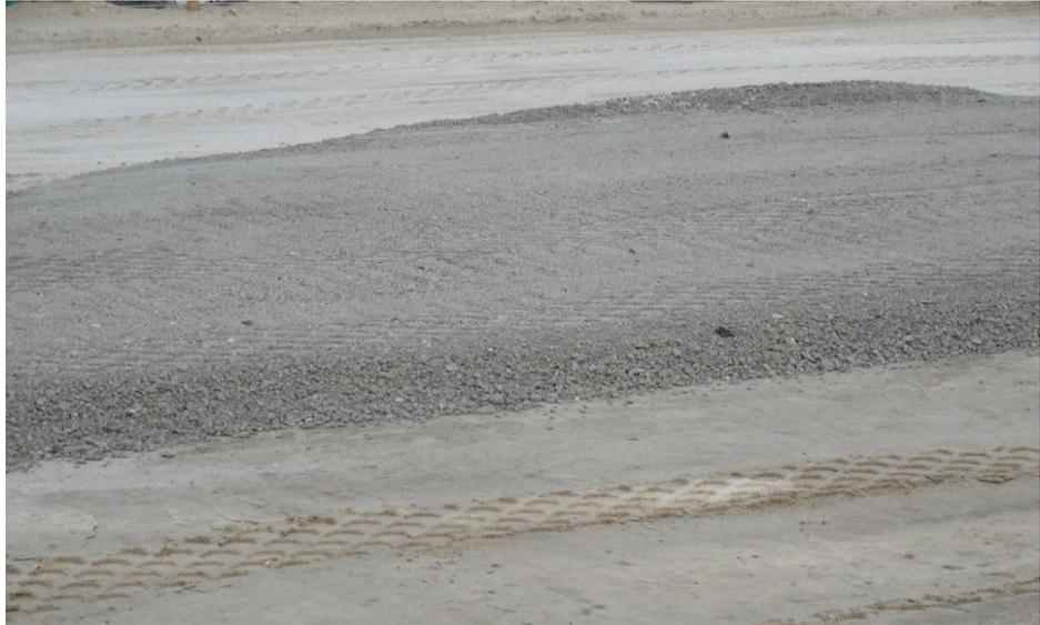
**Figure 5.3:** Project Site #1 I-95 - Photograph of graded aggregate (crushed concrete) used for base under asphalt base
