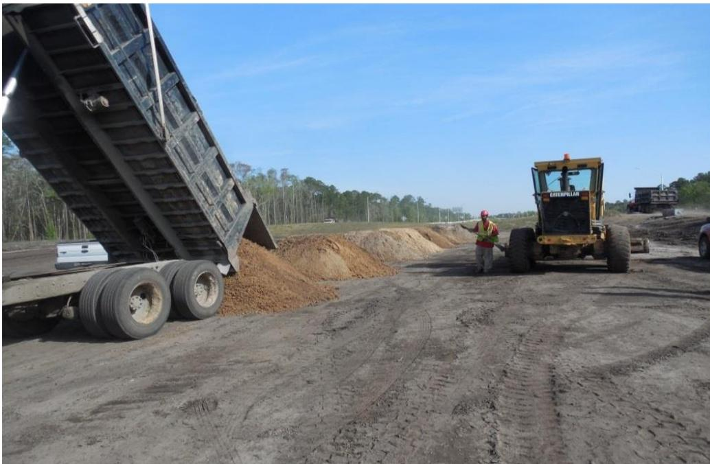
**Figure 5.15:** Project Site #3 SR-9B - Photograph of A-3 embankment material placement
