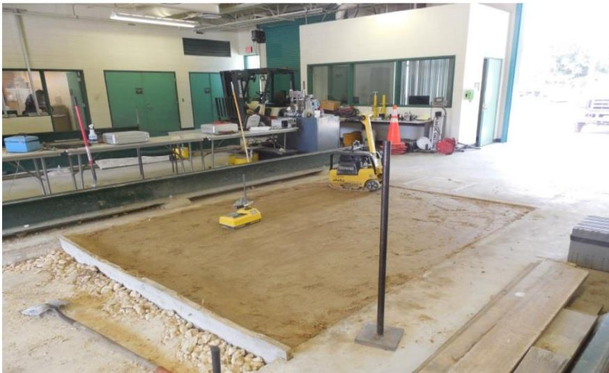
**Figure 4.2:** Photograph of east test pit north stabilized subgrade, NDG for in-place density
