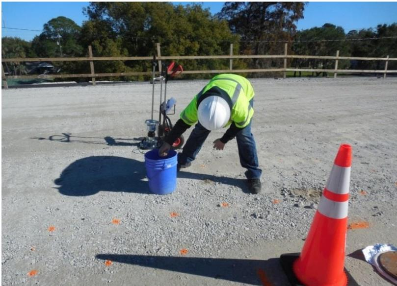
**Figure 5.5:** Project Site #1 I-95 - Photograph of fine sand used as bedding over rough surface texture
