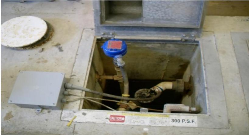
**Figure 3.11:** Photograph of east test pit sump pump (Used to control water level)
