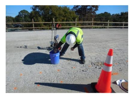
Figure 5.5: Project Site #1 I-95 - Photograph of fine sand used as bedding over rough surface texture
