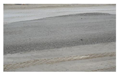
Figure 5.3: Project Site #1 I-95 - Photograph of graded aggregate (crushed concrete) used for base under asphalt base
