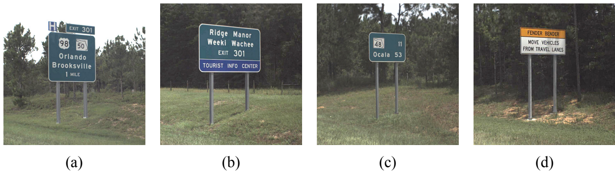
Figure 2.5 Sign structures located along I-75 in Hernando County, FL
