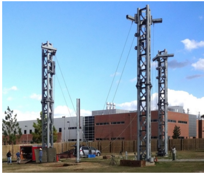
Figure 4.2 High-capacity breakaway connection test article installed at the FDOT pendulum impact test facility (FDOT Structures Research Center, Tallahassee, Florida)
