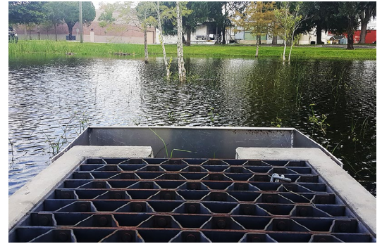
Retention ponds protect Florida groundwater by holding stormwater runoff for a period of time while air and sunlight reduce pollutants.
