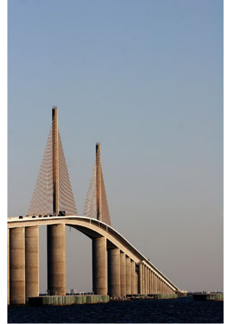
The Sunshine Skyway Bridge, which carries I-275 across Tampa Bay, must be tall enough to allow the largest ocean-going vessels to access Tampa Bay. Notice the pier protection system that prevents off-course vessels or barges from striking the bridge's piers.
