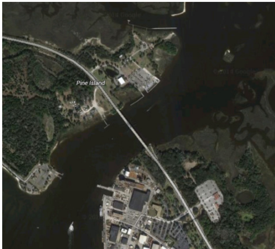
Figure 5.8 Curvature of waterway near Sister's Creek Bridge (Source: Google)
