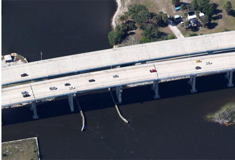
Figure 3.7 Bridge piers protected by land bodies (See lower left and upper right of image; Source: Google)
