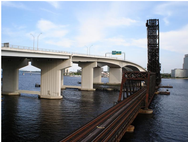
Figure 3.6 Bridge piers protected by adjacent low-rise railroad bridge (Source: https://www.flickr.com )
