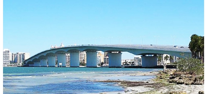
The Ringling Causeway in Sarasota is one of many critical bridges in Florida that employ post-tensioned concrete components.
