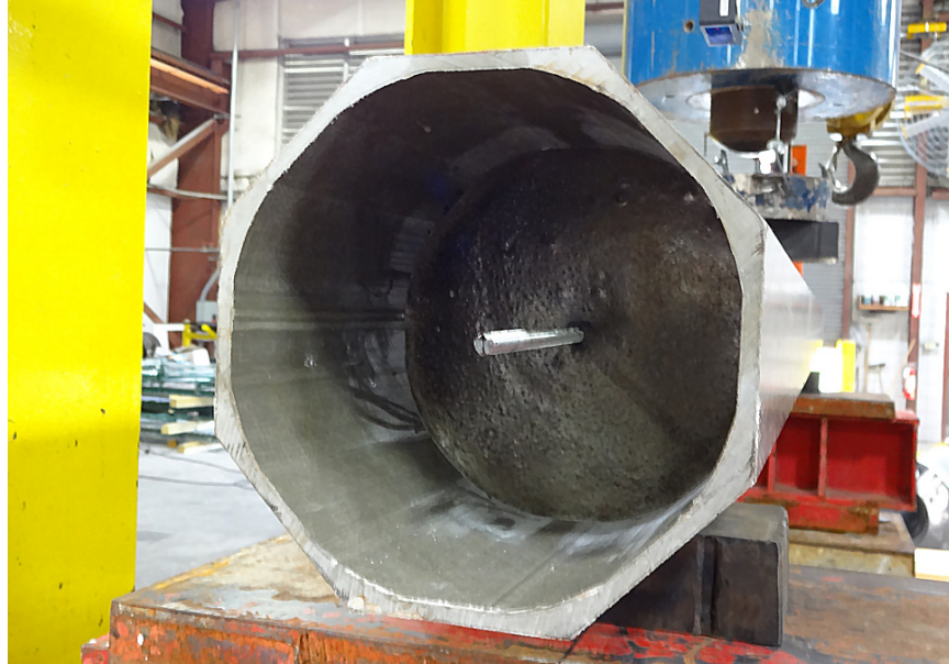
Figure 4.6 Grout plug formed inside FRP post at support point
