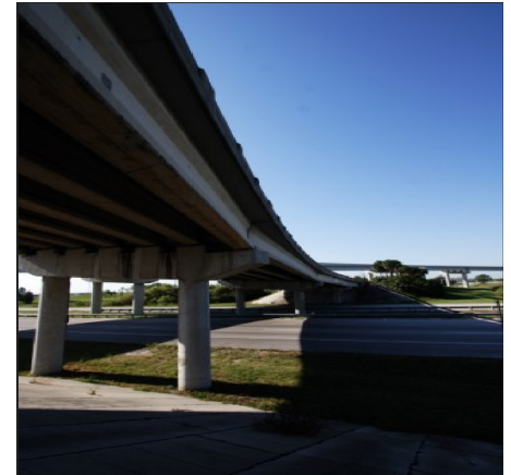
A UF research team updated existing deep foundation software with capabilities to determine spatial variability onsite.
