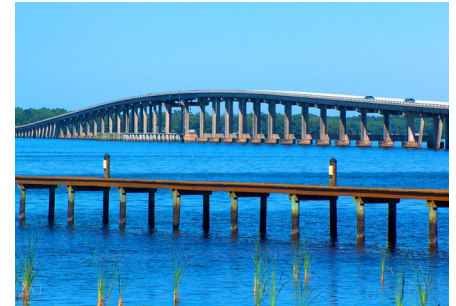
The Shands Bridge (back) at Green Cove Springs is one of many concrete bridges in Florida that replaced wooden bridges (front).
