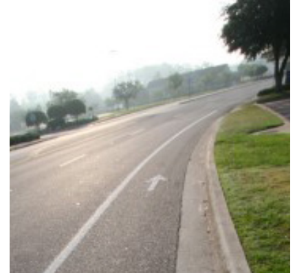
Road departure crashes account for most fatal crashes on horizontal curves like the one seen here. FDOT and University of Florida researchers have developed a database to track high-risk curve locations, resulting in opportunities to enhance curve safety.
