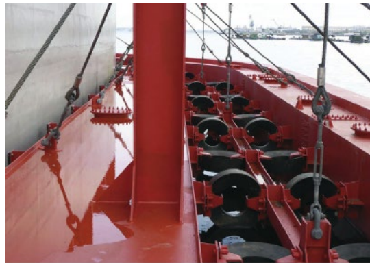
Figure 2.8 Flexible floating protection system installed in Zhanjiang Bay Bridge, China (Wang et al. 2019)
